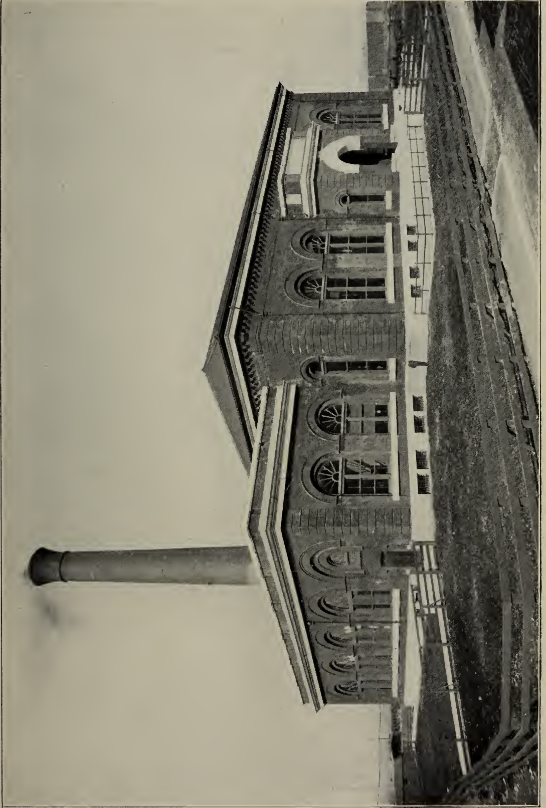
WARD STREET PUMPING STATION.
