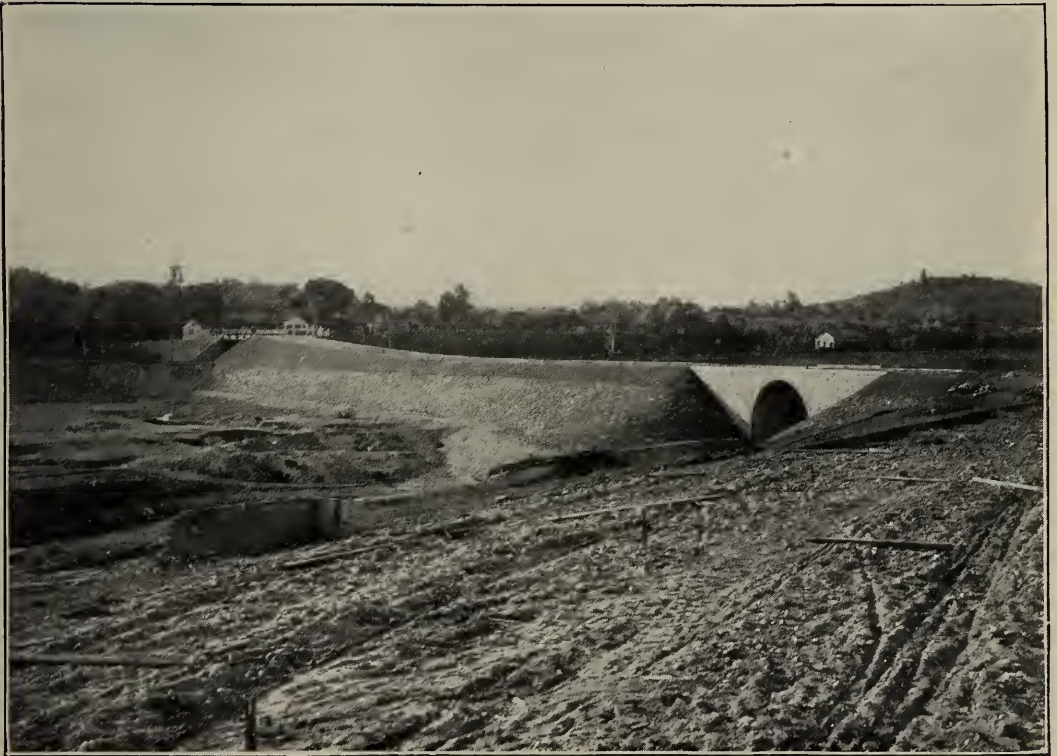
WACHUSETT RESERVOIR—West BOYLSTON MANUFACTURING COMPANY MILLS SITE BEFORE BEGINNING OF WORK AND AFTER STRIPPING OF RESERVOIR AND CONSTRUCTION OF ARCH AND EMBANKMENT.
