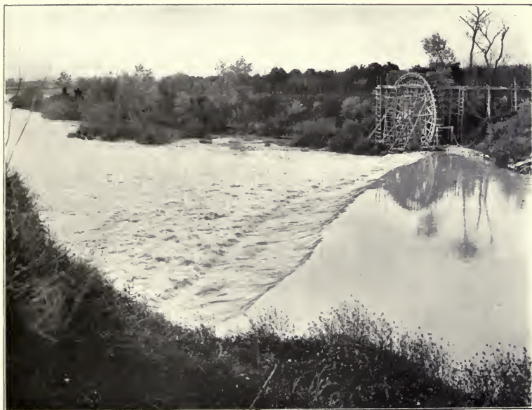
WATER-LIFTING UNDERSHOT WHEEL, SPAIN.
