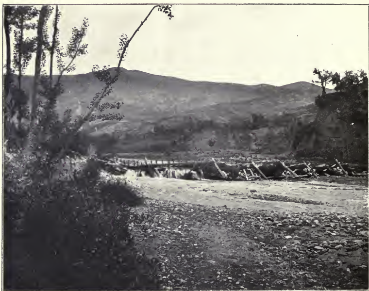
DAM ON THE RIVER GENIL, SPAIN.
