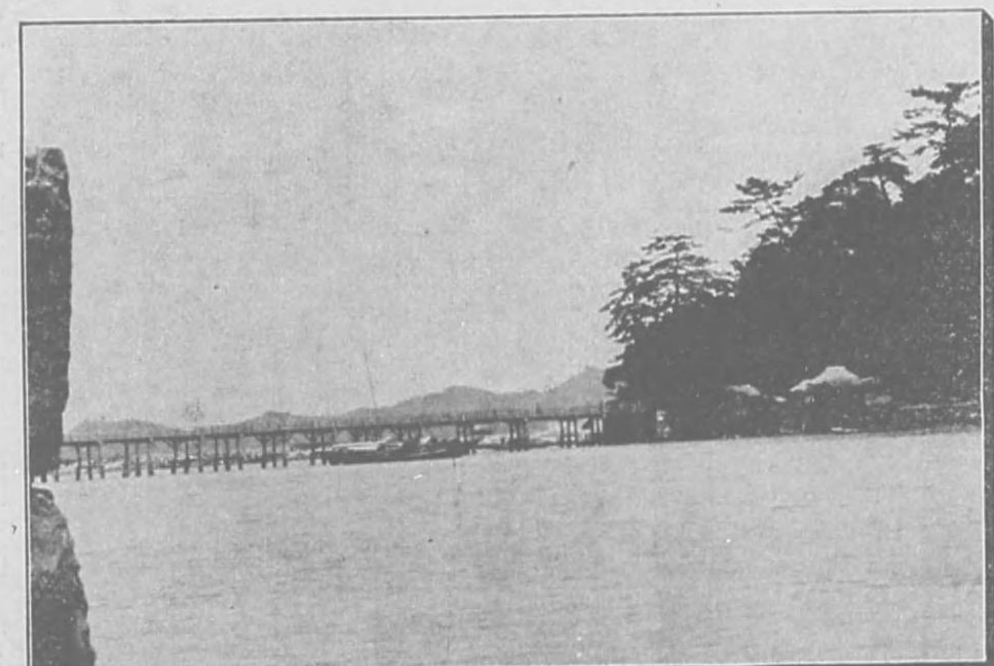
Aoyagi Bridge at Kyūko; Tosa.
