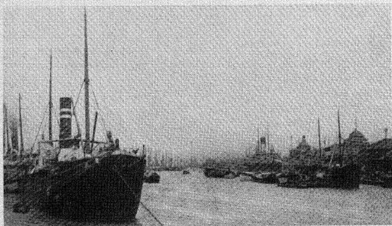
The Old Customhouse located near the Pasig River during the Spanish rule. It is seen at the right with an arch-shaped roof.
