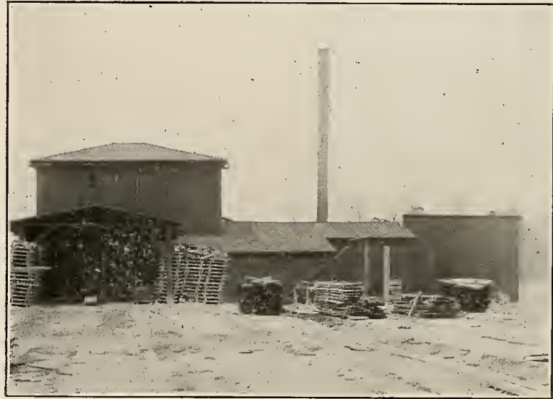
VIEW SHOWING PART OF ROCKY MOUNT BRICK COMPANY'S PLANT
