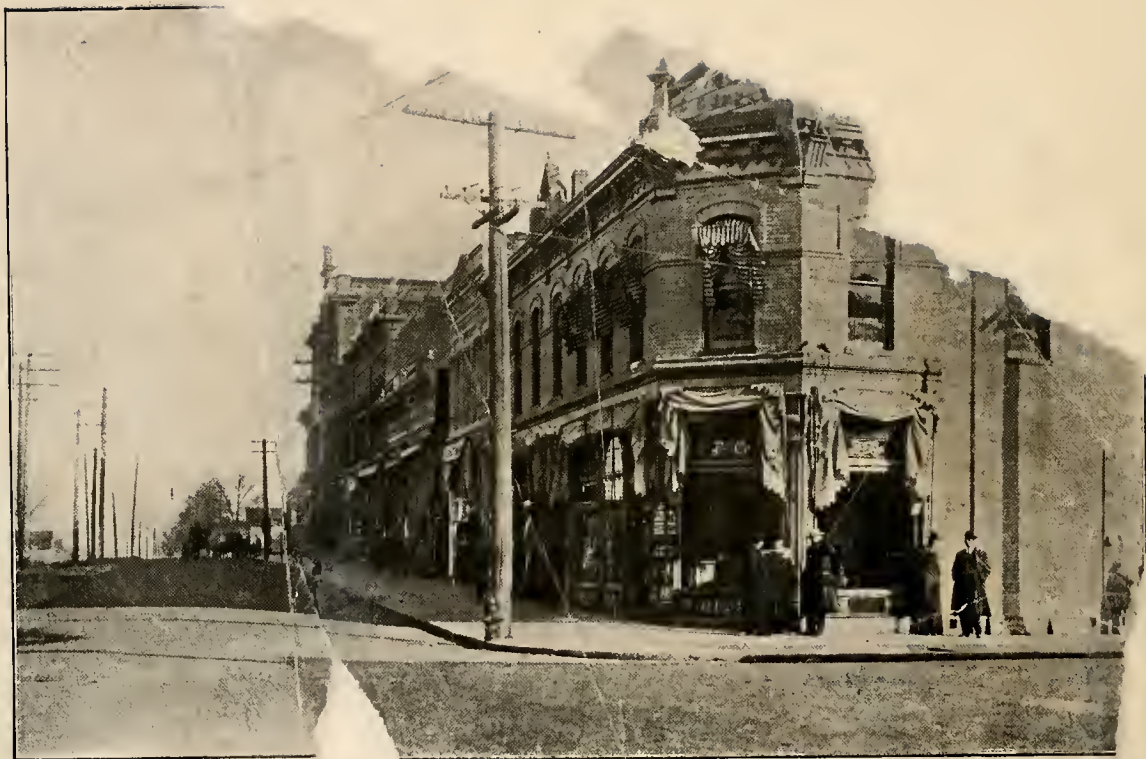
ene Looking North on Main Street.
