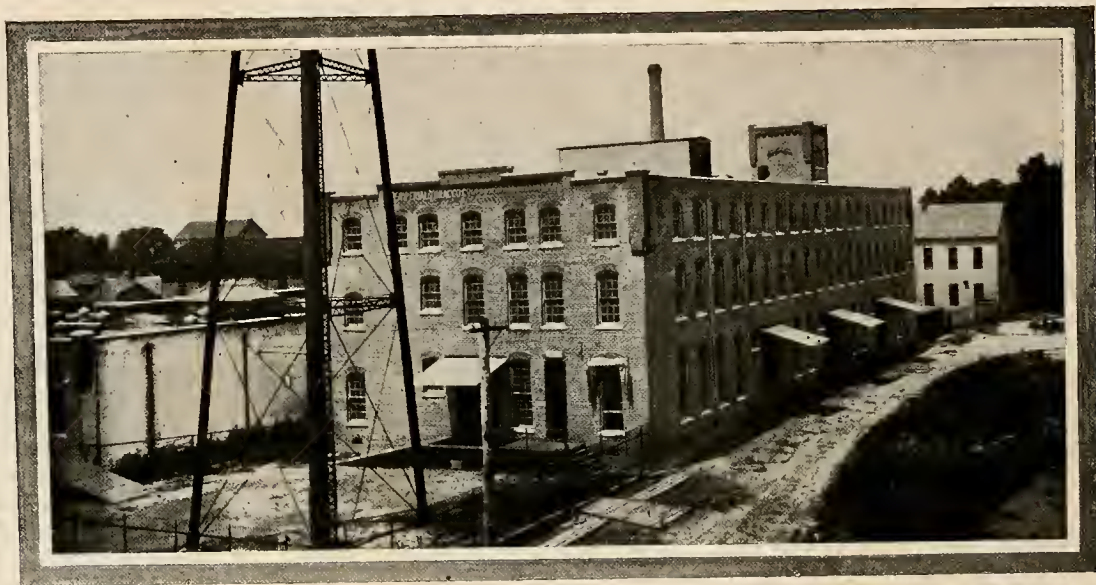
Imperial Tobacco Company's Building, considered Absolutely fire proof and costing nearly $100,000.
