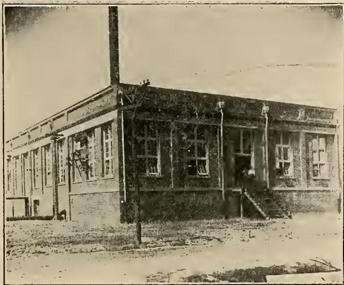
Electric Power and Water Station—Outside View
