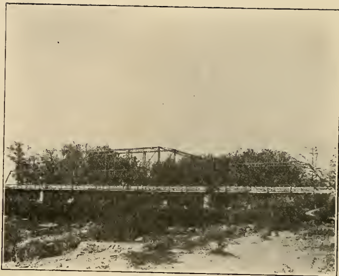
Bridge Over Falls—From A Distance
