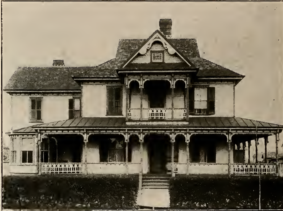
Residence of Mr. W. L. Groom, 226 Franklin Street.
