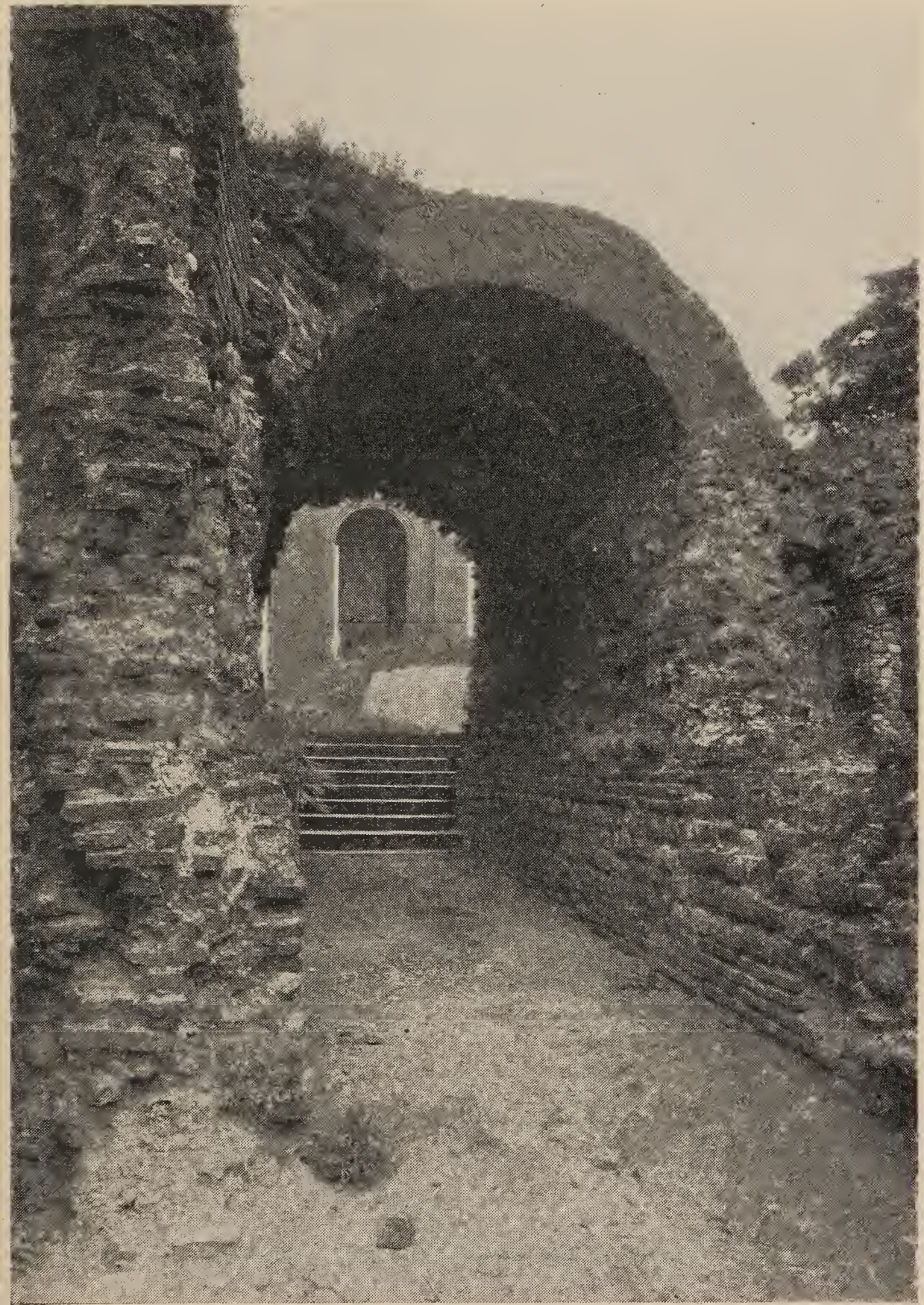
A TOWN GATEWAY Colchester, Balkerne Gate
