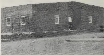
One week later. Siding going up.
