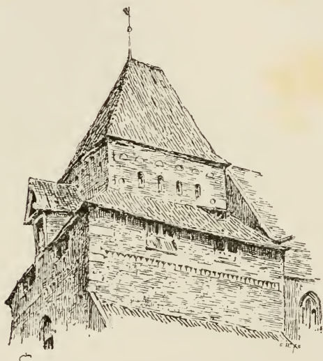
TOWER OF ST. GEORGE'S CHURCH, WISMAR.
