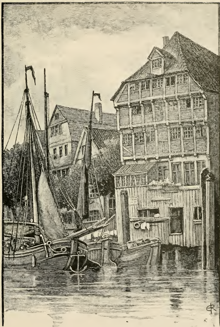
A BIT OF OLD HAMBURG RECENTLY PULLED DOWN.
