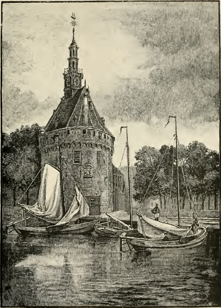
WATER TOWER AT HOORN.
