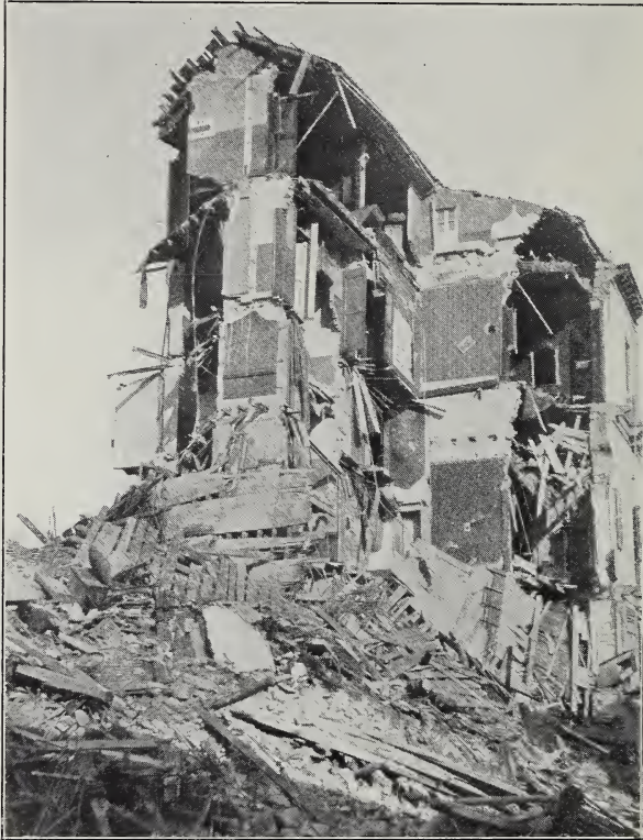
FIG. 13. Wreck of a tall, poorly constructed building.
