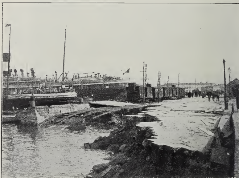
FIG. 3. Collapse of the embankment.
