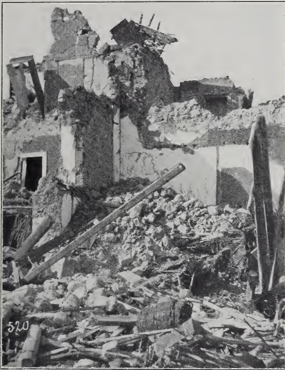
FIG. 6. Showing rubble construction.
