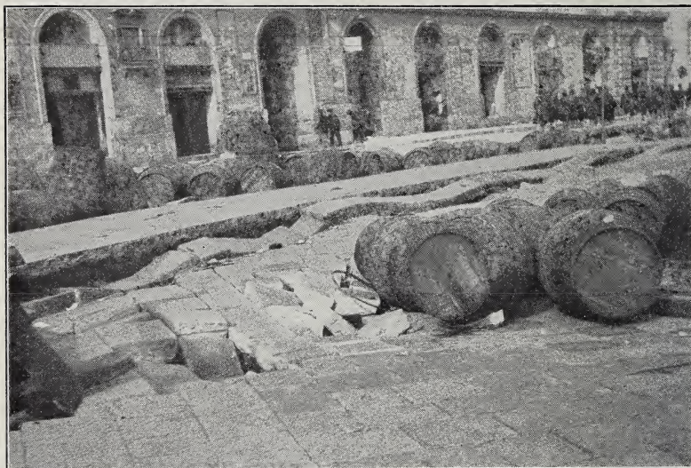
FIG. 5. Free surface wave-forms retained by curb stones of the embankment.
