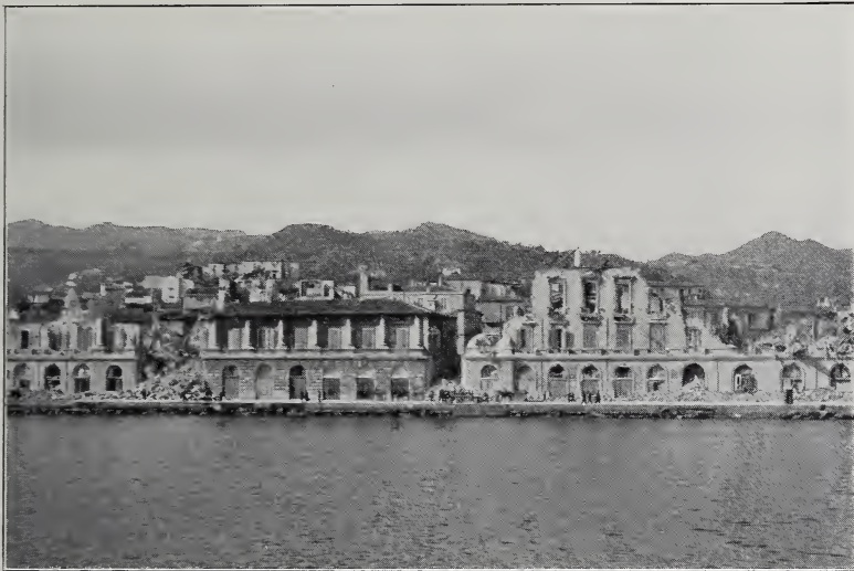
FIG. 2. View along water-front, showing relative stability of low buildings.
