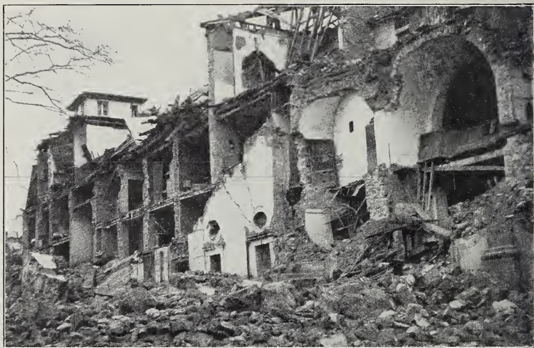
FIG. 11. Fronts fallen from houses, lying East and West.
