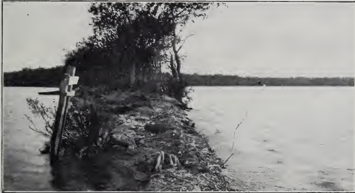
FIG. 3. Partially completed dividing rampart. Lake Detroit.
