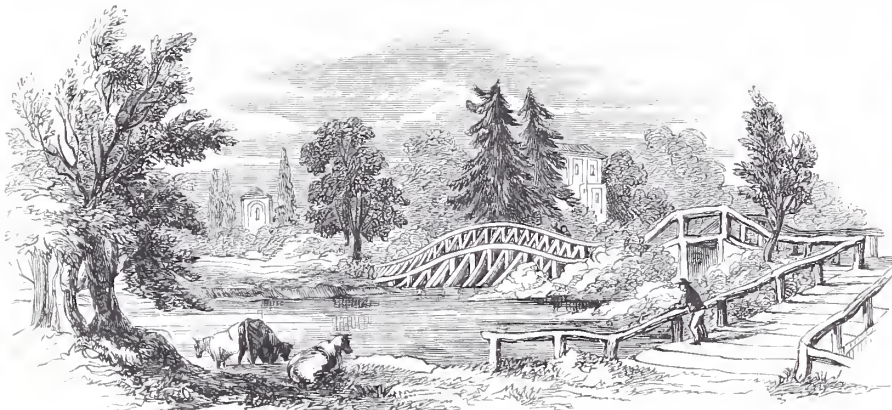
THE WEY BRIDGE.
