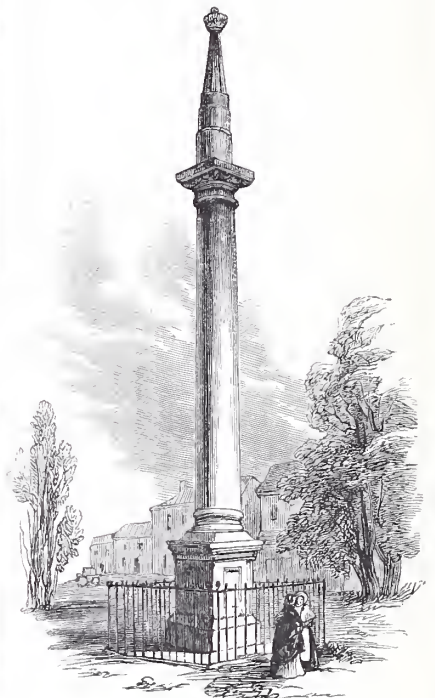
COLUMN AT WEYBRIDGE.
