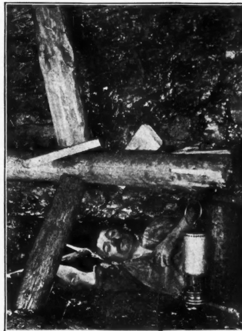
UNDERCUTTING COAL BY HAND.
