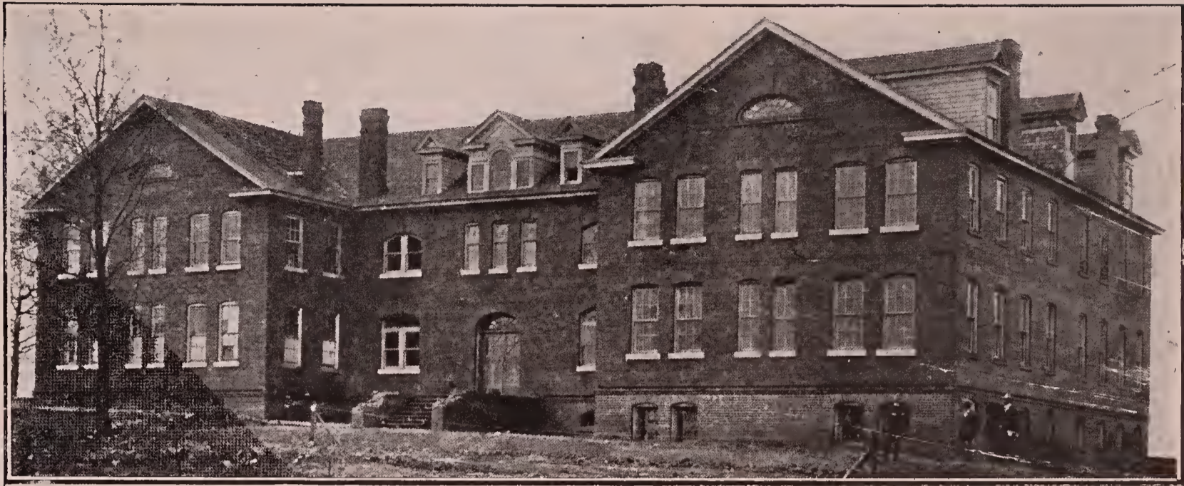
BALLARD INDUSTRIAL BUILDING—LIVINGSTONE COLLEGE
