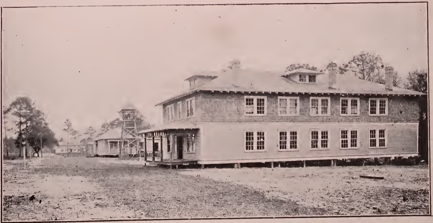
PARTIAL VIEW OF THE NEW HOME OF FLORIDA BAPTIST ACADEMY
