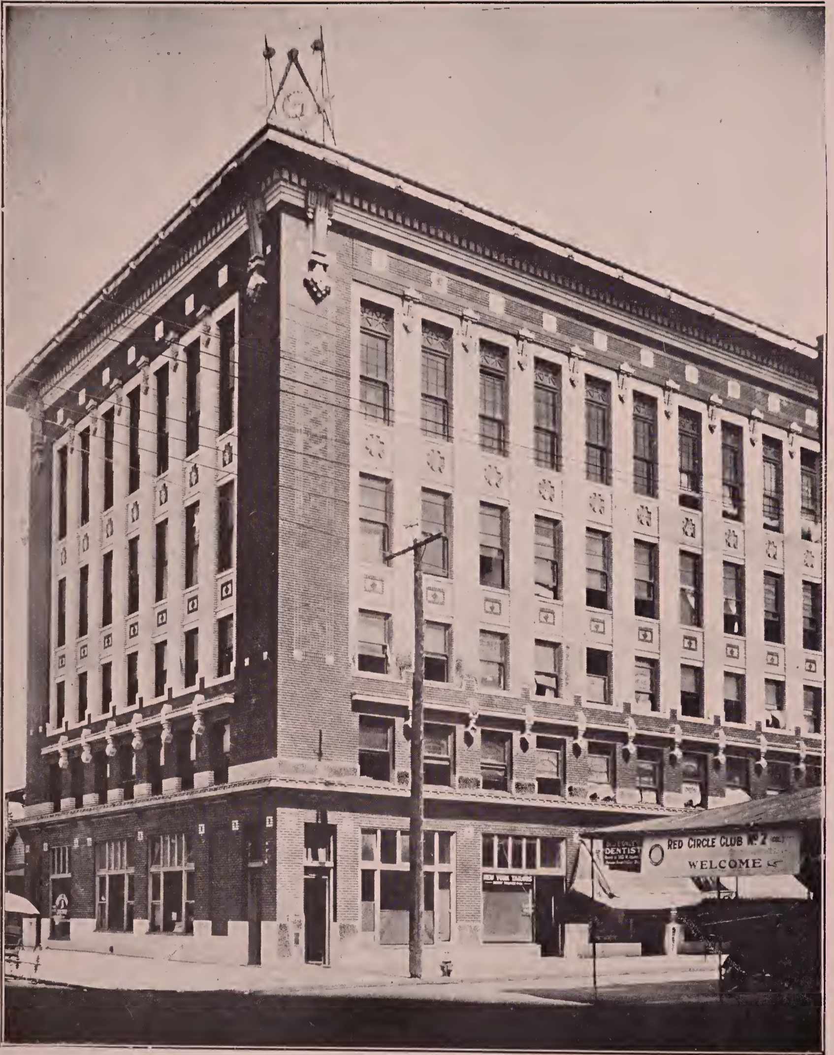
MASONIC TEMPLE BUILDING—JACKSONVILLE, FLA.
