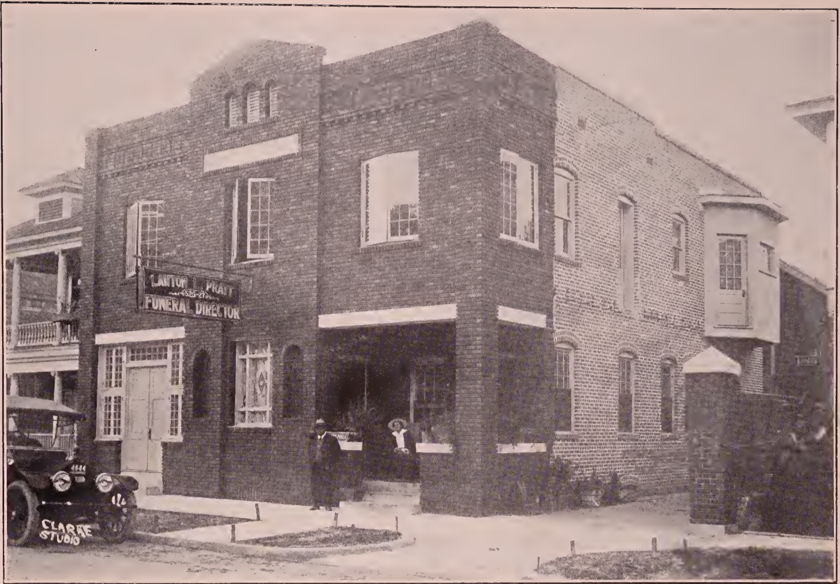
UNDERTAKING ESTABLISHMENT OF L. L. PRATT
