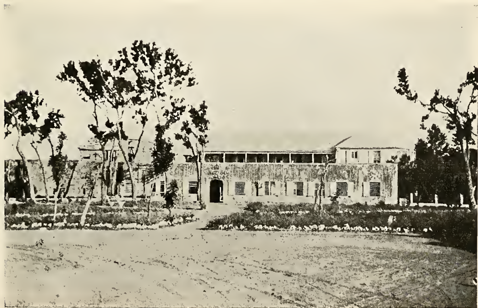
FORT FREDERIKSTED, ST. CROIX
