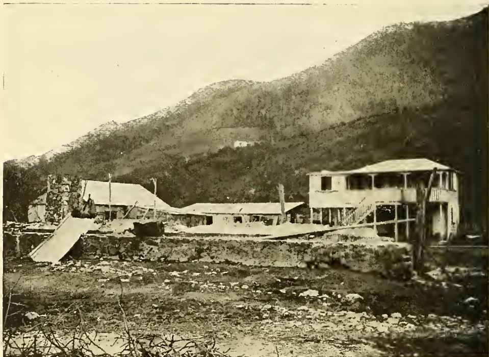
BUILDINGS ON CAROLINE ESTATE, AND BAY-OIL STILL, ST. JOHN
