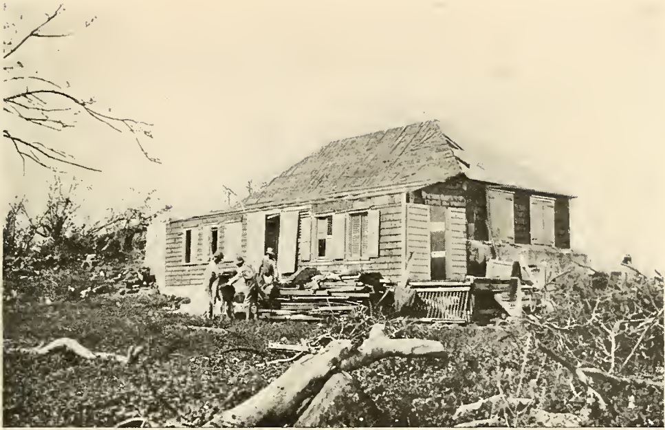
CANAAN ESTATE HOUSE, AFTER HURRICANE
