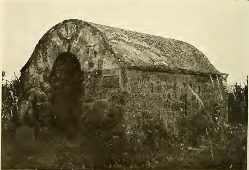
TYPICAL OLD WATCH HOUSE ON SUGAR ESTATE, ST. CROIX
