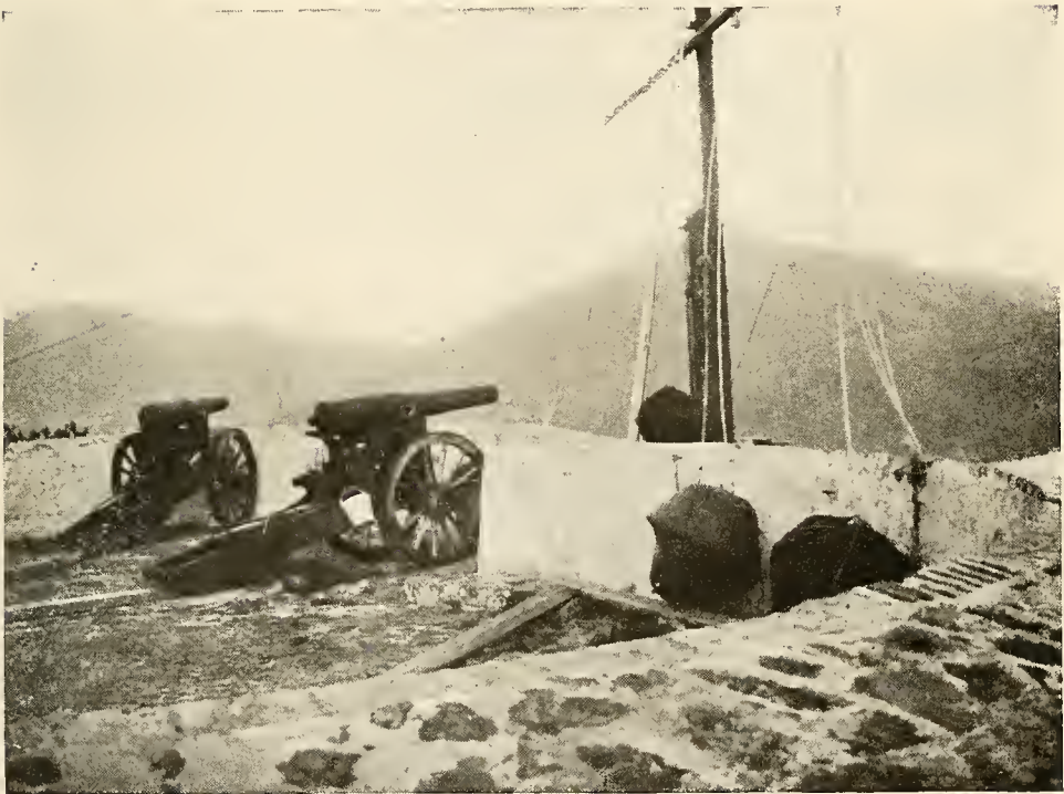
SIGNAL STATION, TOP OF COWELL'S BATTERY
