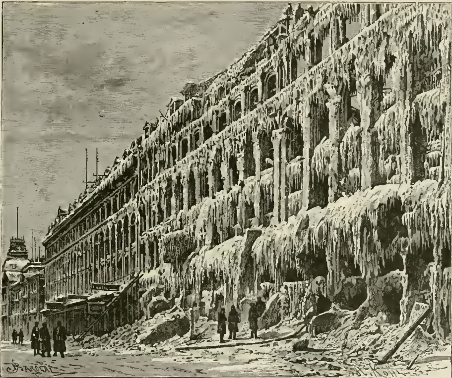
Fig. 140.—ICICLES ON THE FRONT OF A HOUSE AFTER A FIRE.
