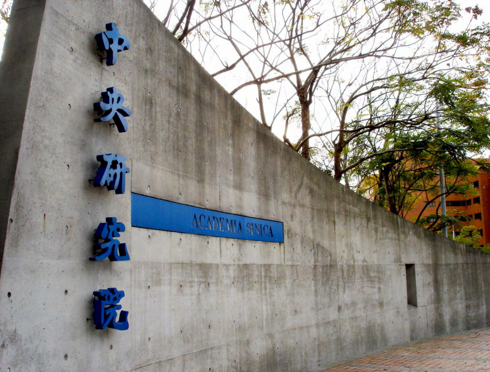
The wall beside the gate of Academia Sinica.
