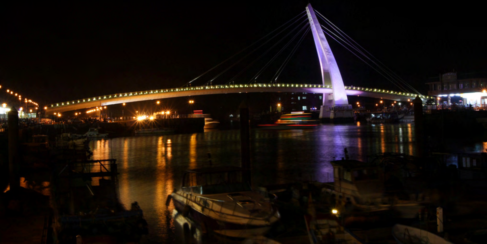
■ Lover Bridge of Tamsui
