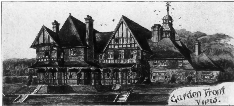
House at Broxbourne, DUDLEY NEWMAN, F.R.I.B.A., Architect.
