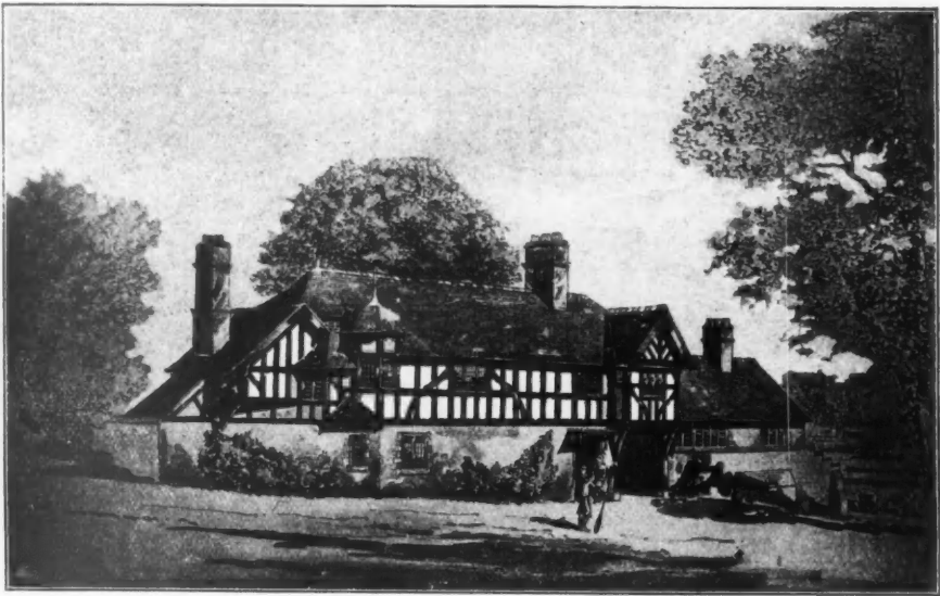
New Premises for the Chester Boat Company, Ltd., THOS. M. LOCKWOOD AND SONS, Architects.
