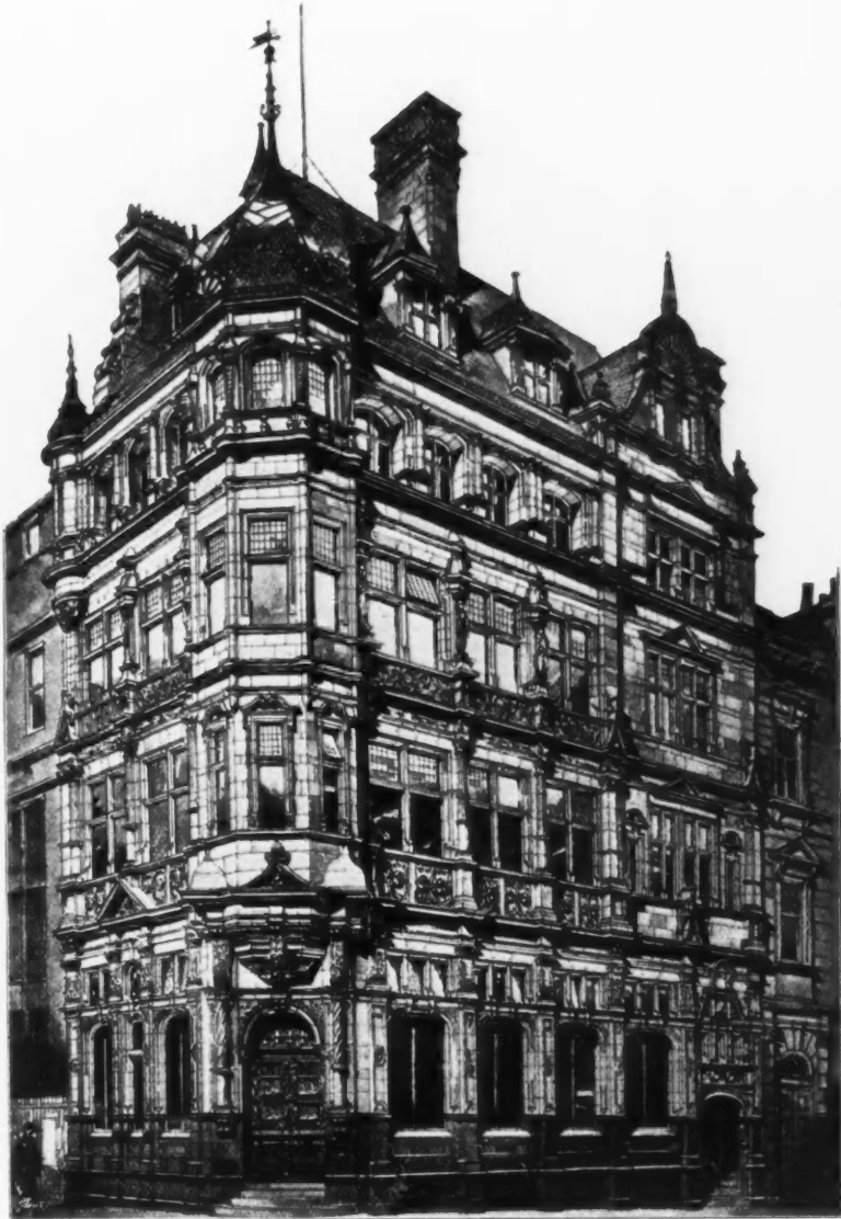
Adelphi Bank, Liverpool, W. D. CARÖE, M.A., Architect.
