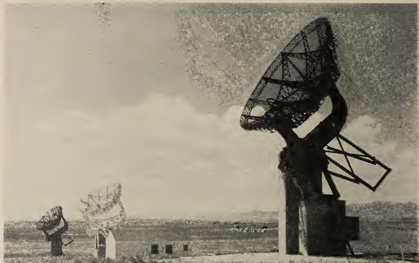
Radio telescopes installed at Gunbarrel Hill, near Boulder, Colorado, for measuring radio noise reaching the earth from the sun and outer space. Such phenomena affect communication and radio navigation service in the VHF range.
