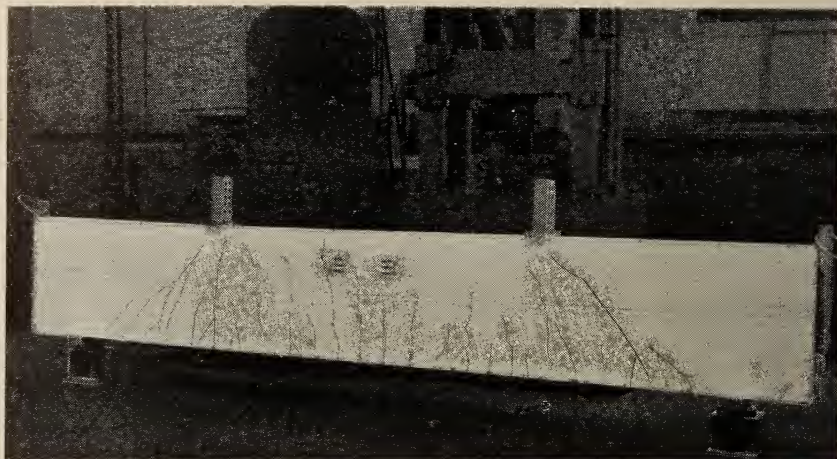
Typical crack pattern at failure of a loaded reinforced concrete beam. Many such tests were performed in a study of the cracking of reinforced concrete.
