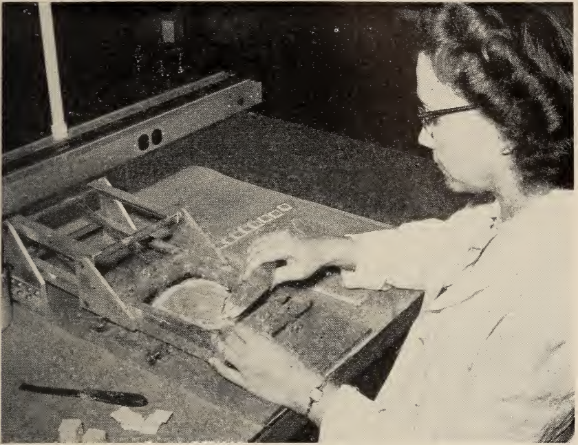
A step in the making of tape capacitors for the mechanized production of electronics program (p. 18).
