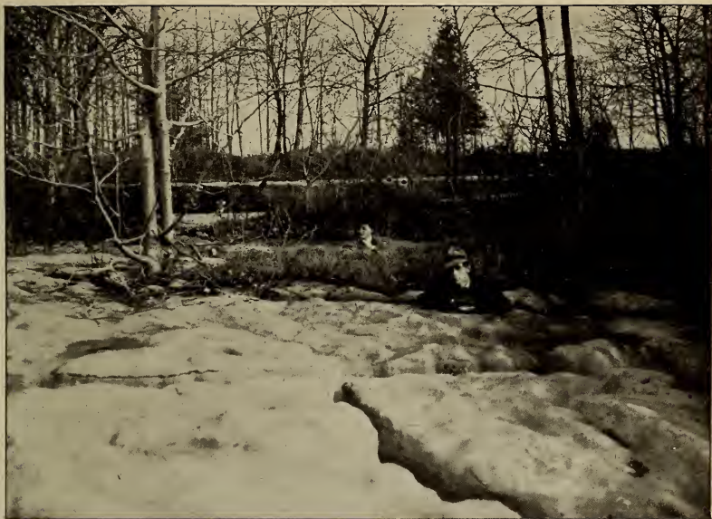
The Karsten , showing effect of surface and ground water on Onondaga limestone. The water dissolves the rock along the joint planes forming deep fissures which widen into caves in places. Some of these fissures extend to a depth of 100 feet or more. On top of cliff at Blue lake
