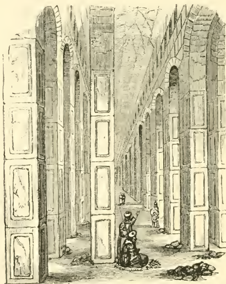
Underground Buildings in the south-east corner of the Haram es Sherif.
