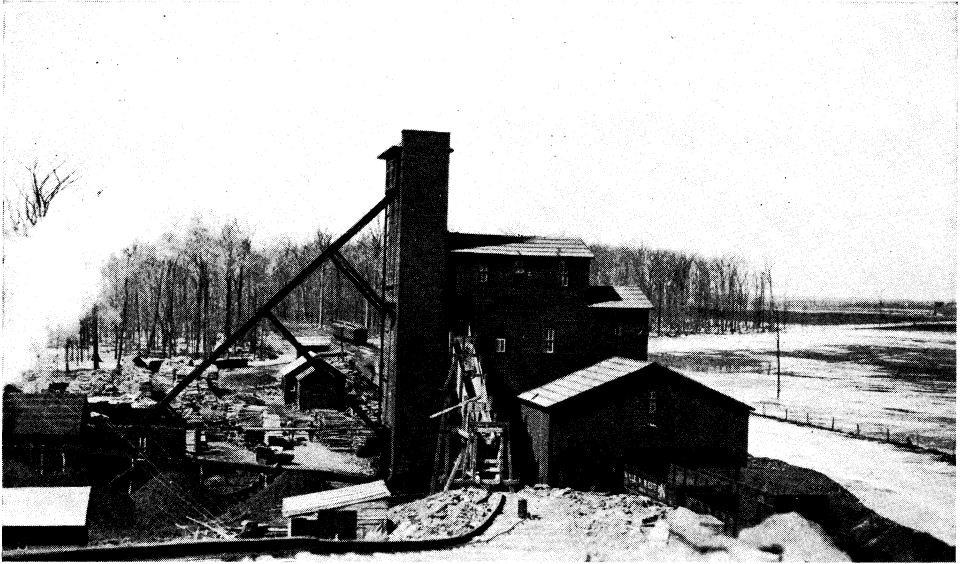
TIPPLE OF BLISS COAL MINE, SWAN CREEK
