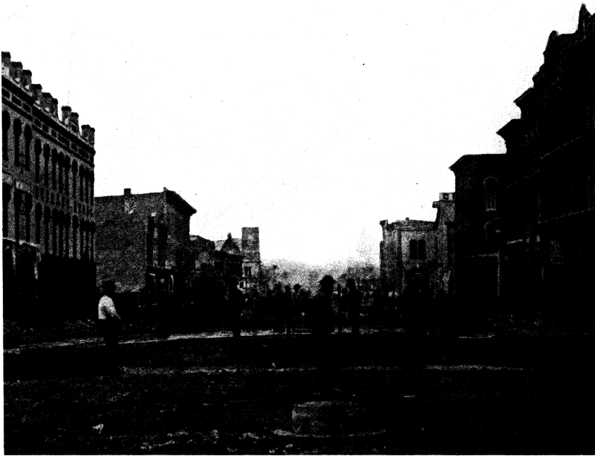
LAYING NICHOLSON PAVEMENT IN GENESEE STREET, 1868
