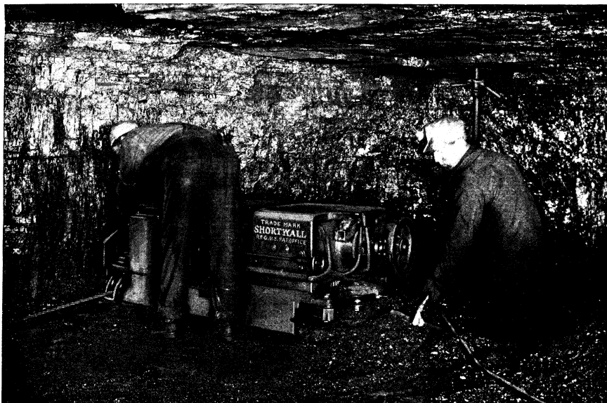
CLOSE UP VIEW OF SHORT WALL CUTTER, SHOWING COMPACTNESS OF CONSTRUCTION
