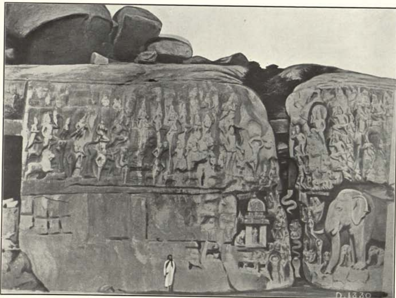
(a) GENERAL VIEW, BEFORE REPAIRS.
