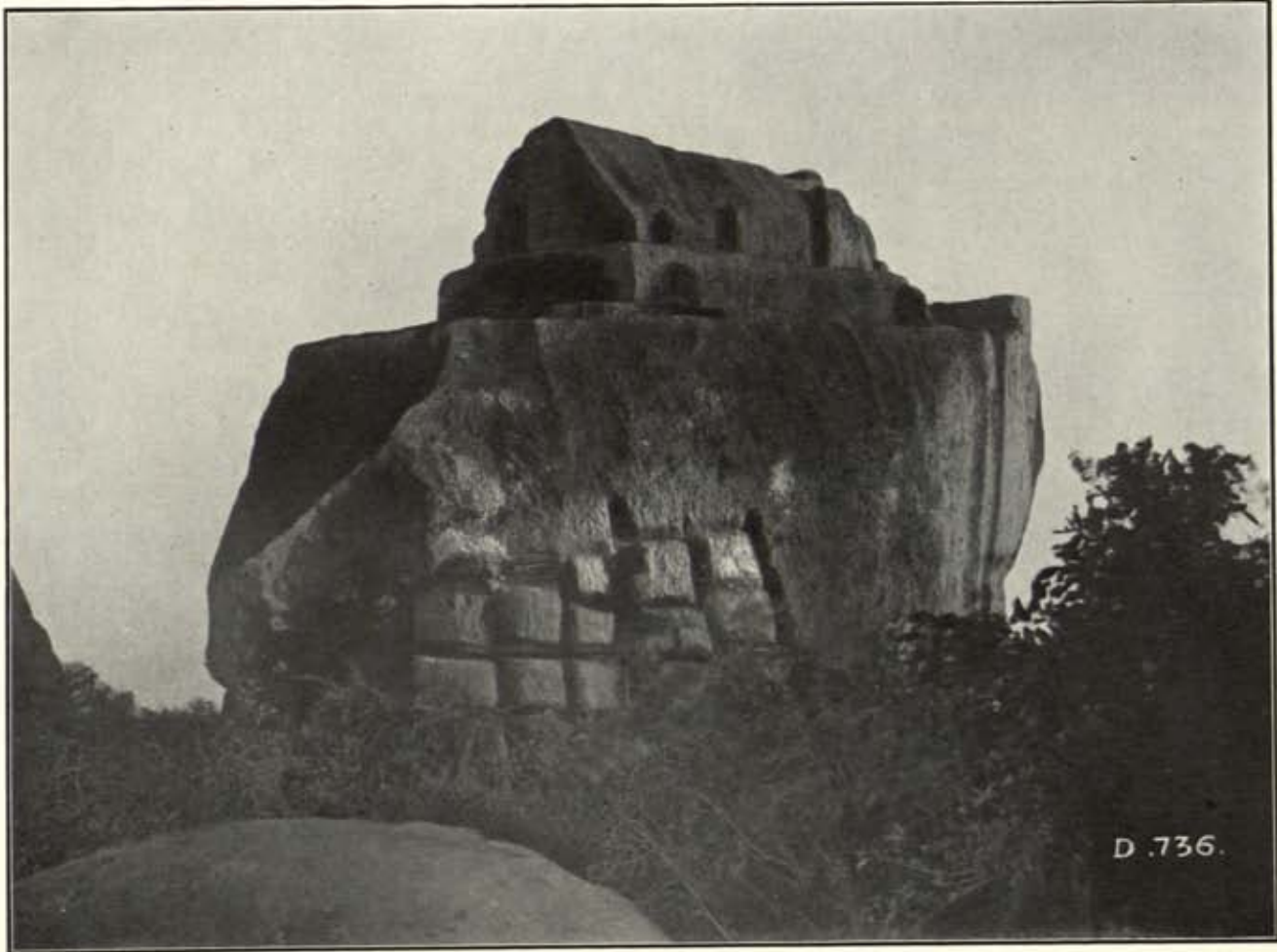
(a) METHOD OF EXCAVATING A RATHA.
