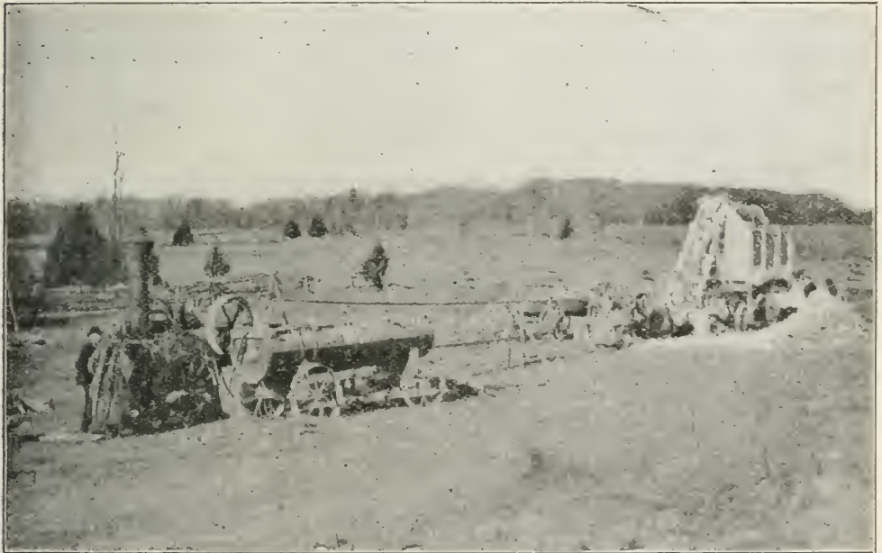
Crushing Stone for Lanark County Roads.
