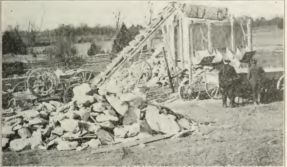
Crushing Stone for Lanark County Roads.
