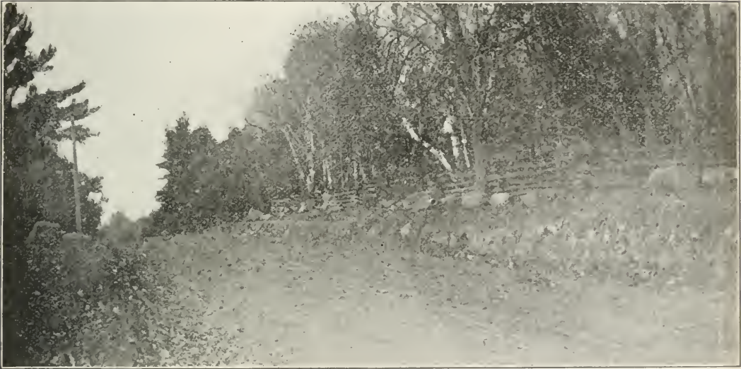
Good work with a Grader - near Orillia.
