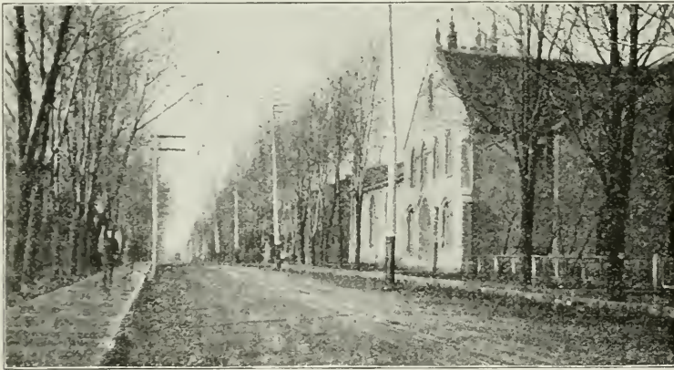
Sidewalk outside of Trees and the Roadway Narrowed.
