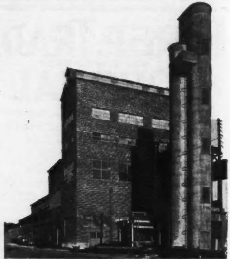
A Typical Austin Unit Responsibility operation. The Columbia River Paper Mill, Vancouver, Wash. Designed, built and equipped by Austin.
