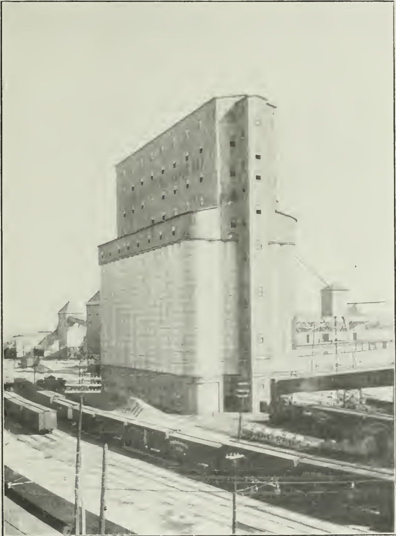
MONTREAL HARBOUR — HARBOUR COMMISSIONERS' ELEVATOR — BUILT 1903.
