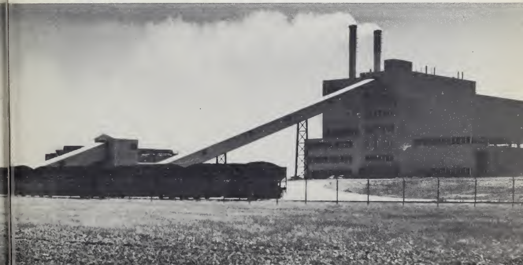
Central's steam plant at Minot, N. Dak., uses lignite for fuel.
