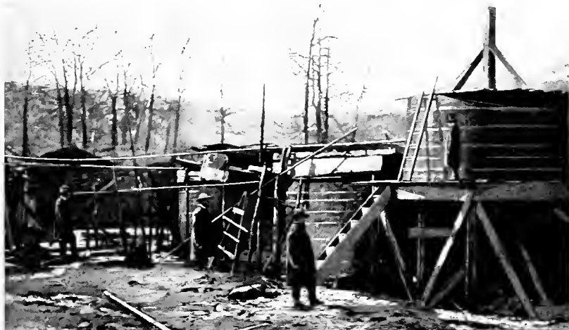
WOODEN TANKS FOR STORING OIL
