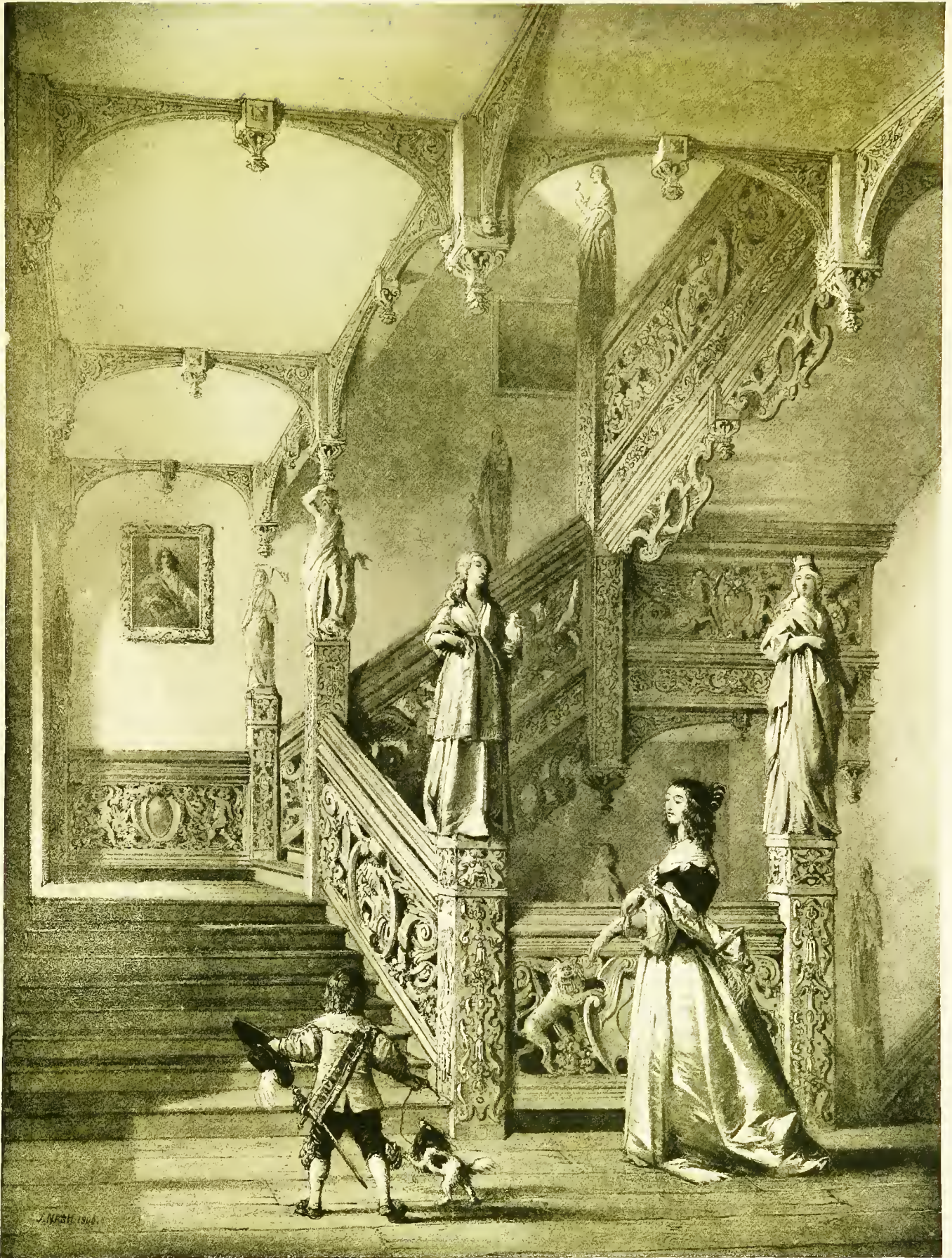
ALDERMASTON, BERKSHIRE: THE STAIRCASE.
