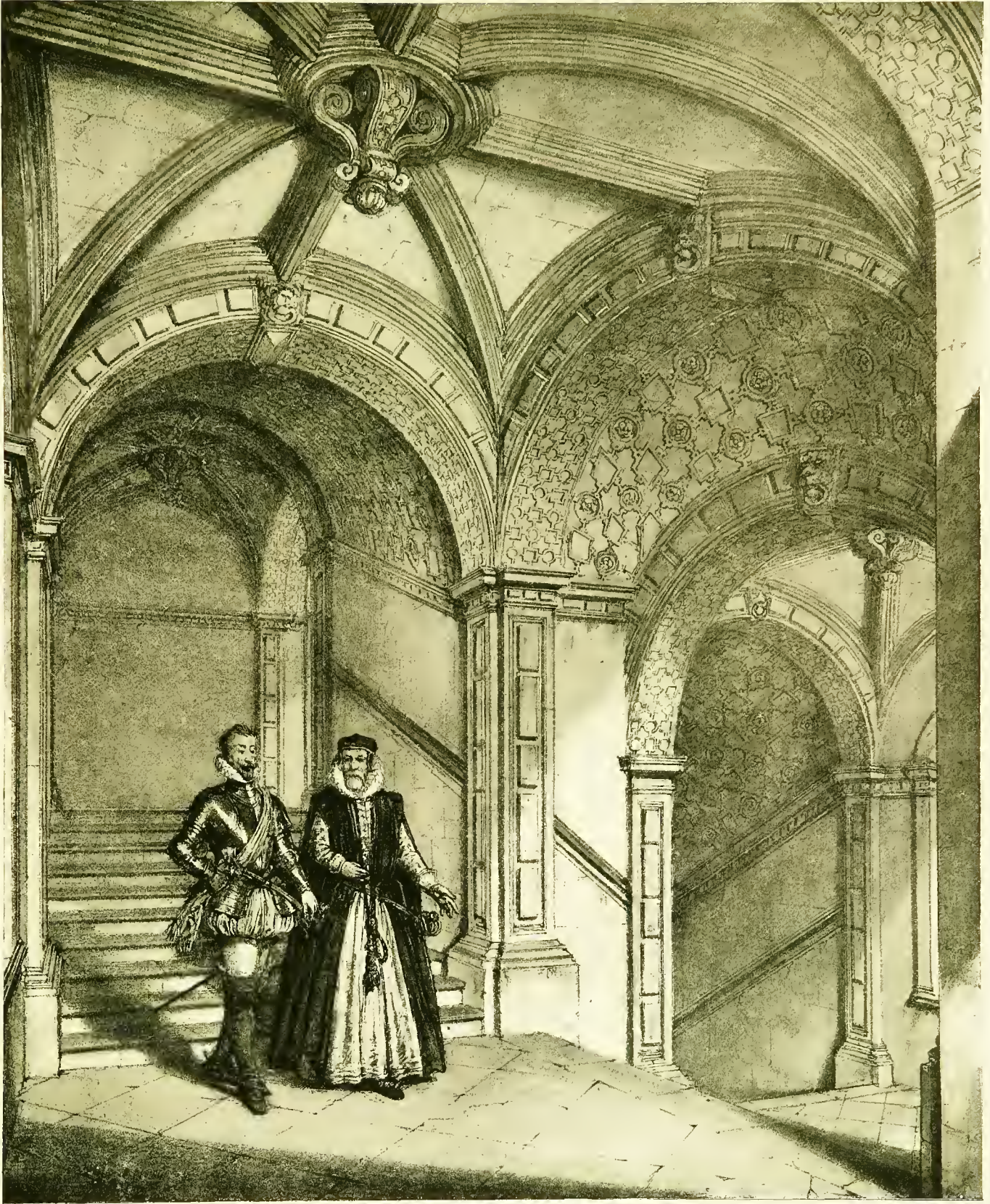
BURLEIGH, NORTHAMPTONSHIRE: THE STAIRCASE.
