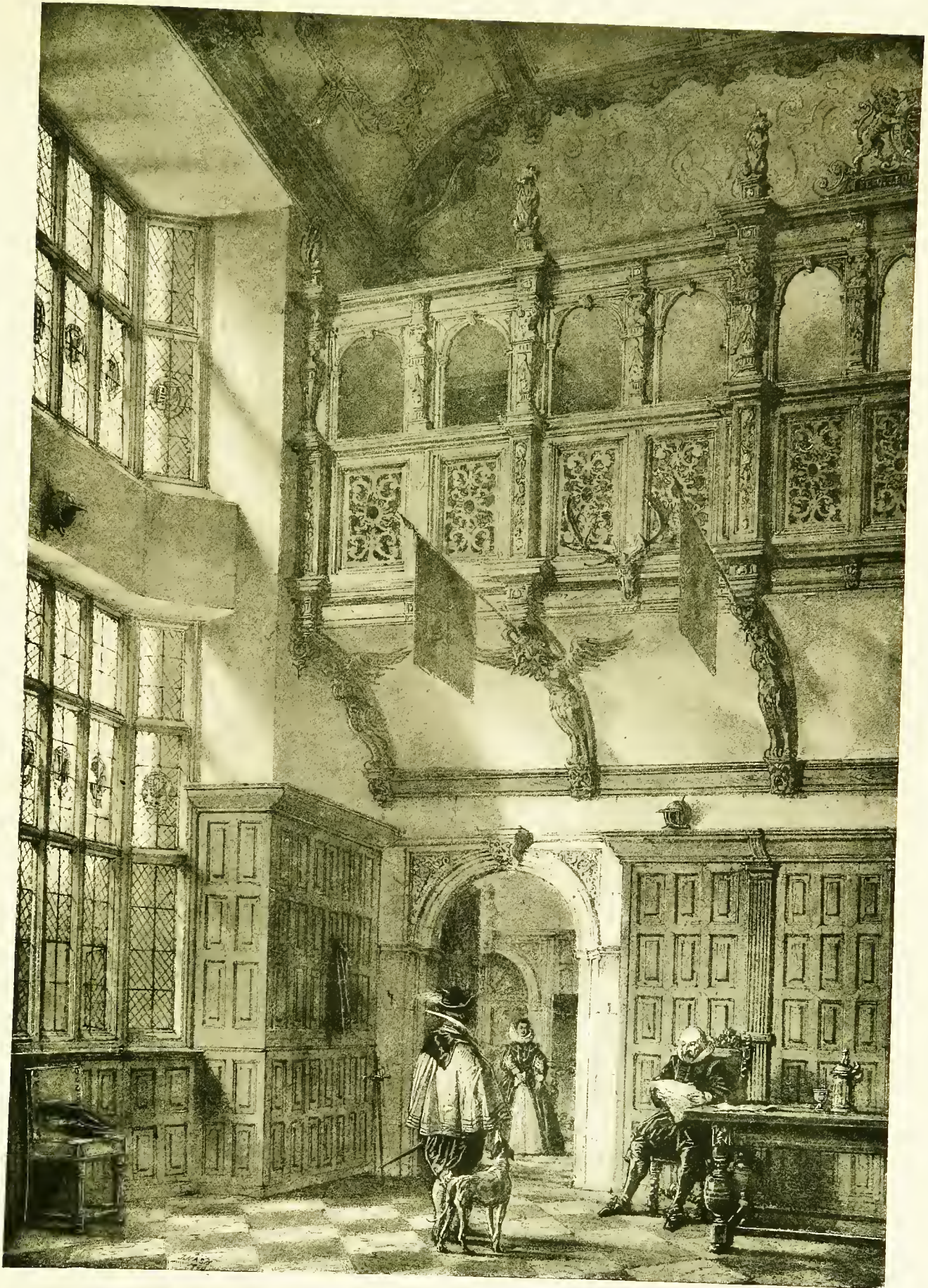
HATFIELD HOUSE, HERTFORDSHIRE: GALLERY IN THE HALL.
