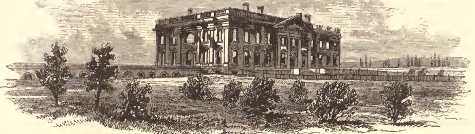
REMAINS OF THE PRESIDENT'S HOUSE AFTER THE FIRE.
