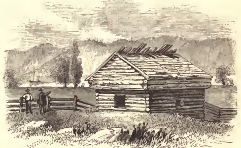
BLOCK-HOUSE AT NORTH BEND. 4
