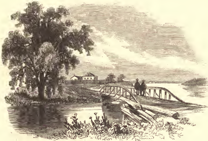
STREET'S CREEK BRIDGE, LOOKING NORTH. 1
