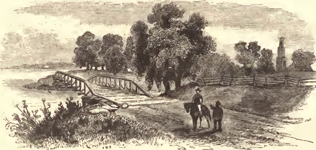
STREET'S CREEK BRIDGE. 1
