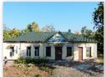
Shyrokyi Railway Crossing Loop 2018 01.jpg
