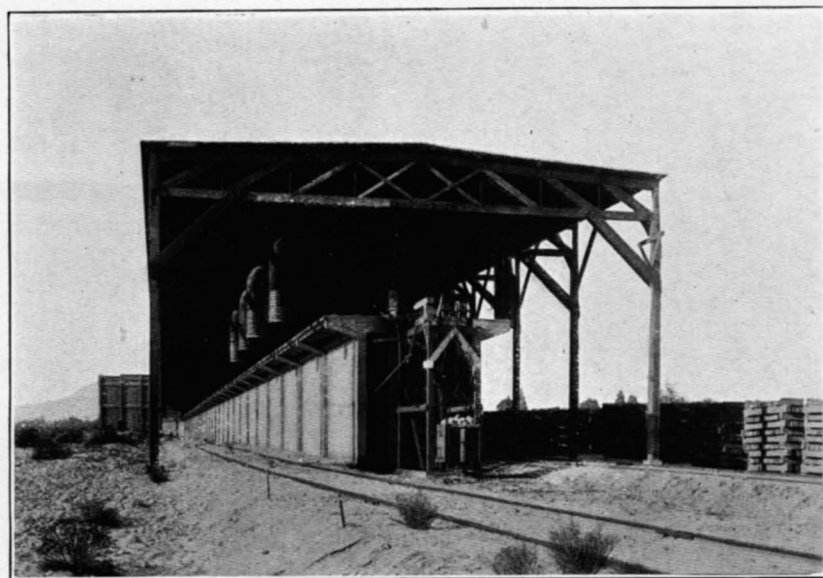
FIG. 2.—END VIEW OF PRECOOLING SHED.
