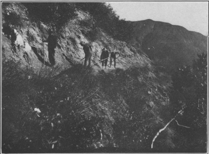
FIG. 2.—GRADING IN A MOUNTAIN TRAIL IN A ROUGH PLACE.
