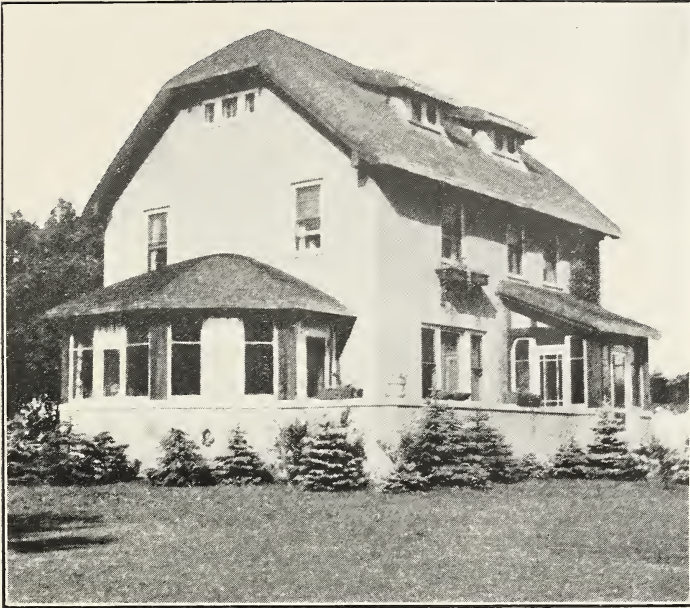
FOUNDATION PLANTING OF EVERGREENS
