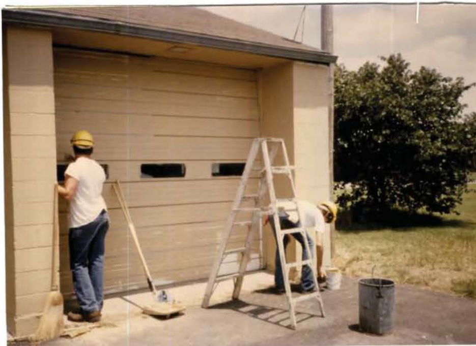
YCC painted the old office/shop complex to match the new. (WRJ)
