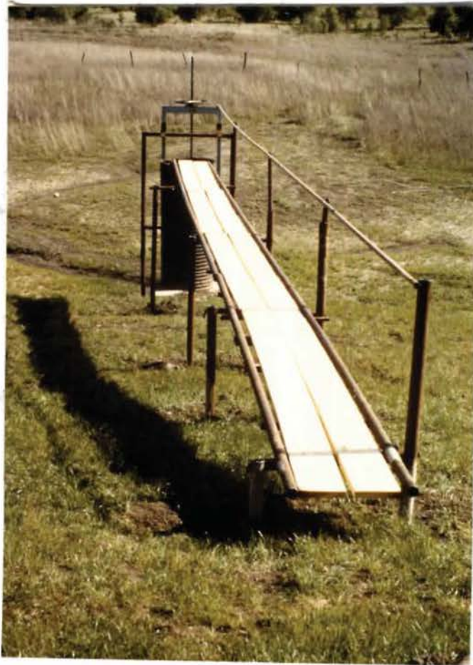
Final Rehabilitation of Elm Pond WCS- construction of a walkway. (WRJ)
