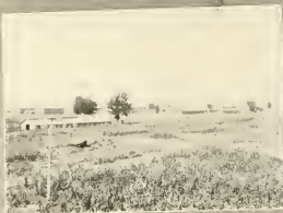
STABLES UNDER CONSTRUCTION
