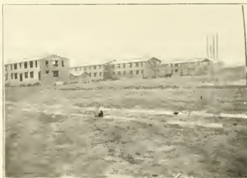
BUILDING ADDITIONS TO THE REGIMENTAL BARRACKS
