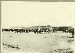
DRILL OF BATTERY MOUNTED
