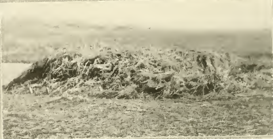
CAMOUFLAGED ROOF AND ENTRANCE TO TELEPHONE DUGOUT, 331ST F. A.
