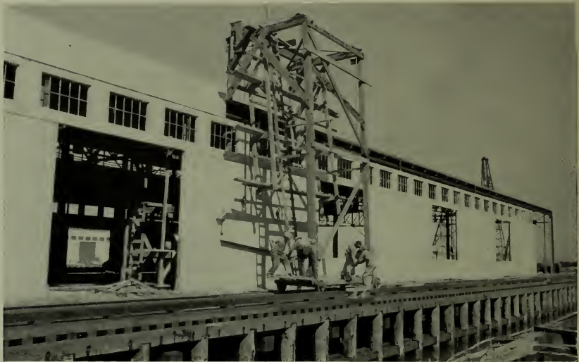
INSTALLATION OF PRECAST REINFORCED CONCRETE WALL SLABS, TRANSIT SHED, PIER 19
