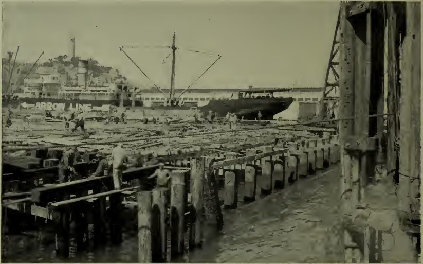
SUBSTRUCTURE OF PIER 9 UNDER CONSTRUCTION
