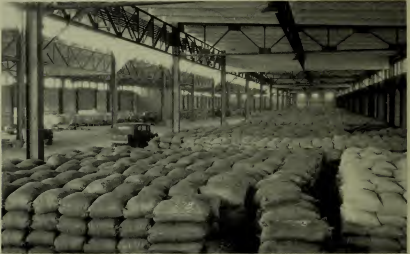
TYPICAL CARGO SCENE OF INTERIOR OF ONE OF THE HUGE TRANSIT SHEDS AT PIER 45
