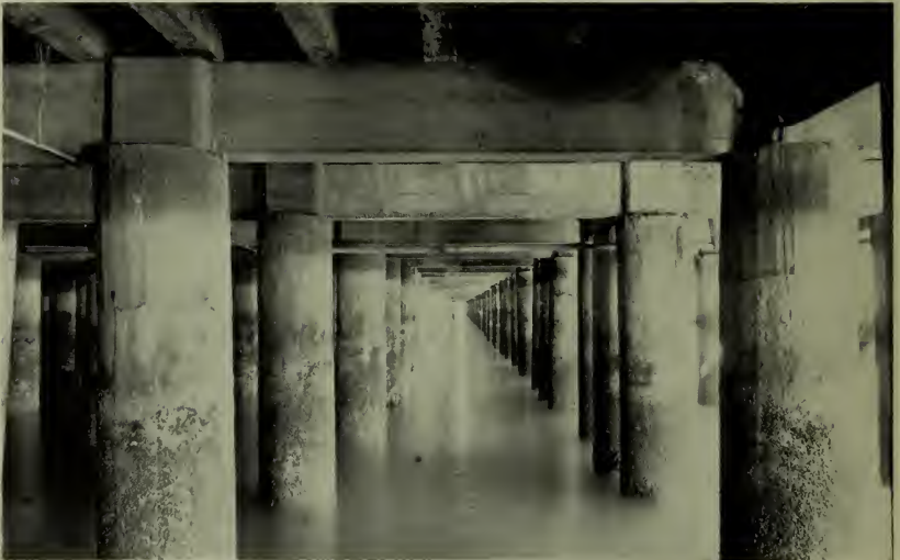
PRECAST REINFORCED CONCRETE PILE JACKETS INSTALLED IN 1912—IN PERFECT CONDITION AFTER TWENTY-SIX YEARS EXPOSURE TO SEA WATER.
