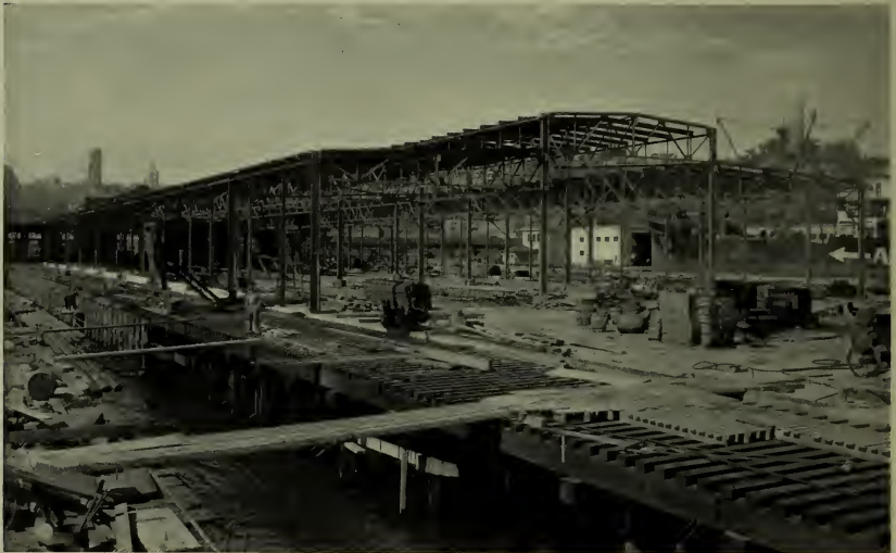
STEEL FRAME TRANSIT SHED ON PIER 9 UNDER CONSTRUCTION
