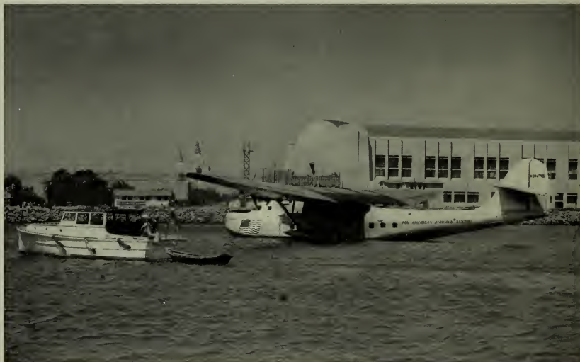
GENERAL VIEW OF HANGAR B, ONE OF TWO SUCH STRUCTURES COMPLETED AT TREASURE ISLAND AT A COST OF $450,000 EACH
