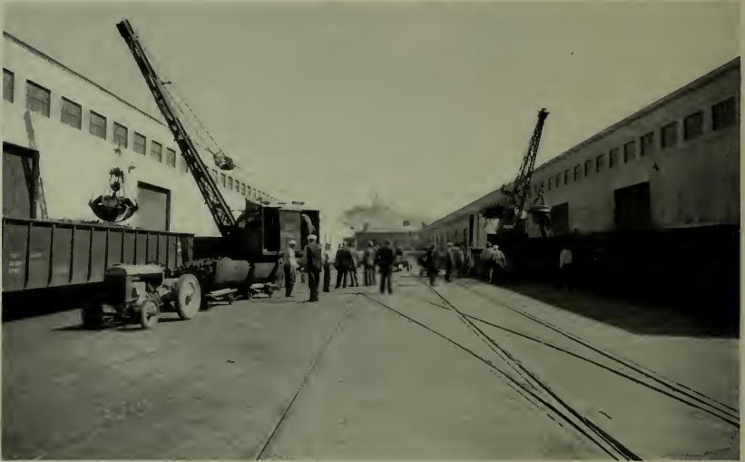
VIEW OF AREA BETWEEN SHEDS A AND B, PIER 45, WITH TELEGRAPH HILL IN BACKGROUND— UNLOADING SCRAP IRON FOR TRANSSHIPMENT
