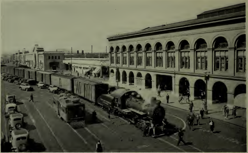
THE STATE BELT RAILROAD IS AN OUTSTANDING HARBOR FACILITY—VIEW OF FREIGHT MOVEMENT ON THE EMBARCADERO
