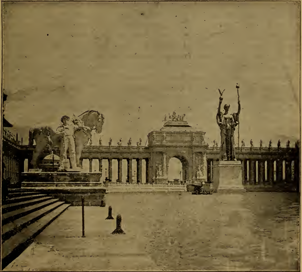
ENTRANCE TO BASIN.
