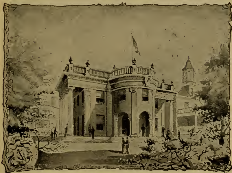
RHODE ISLAND BUILDING.
