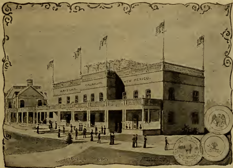
JOINT TERRITORIAL BUILDING.
