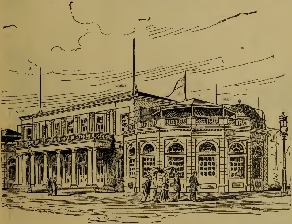
PUBLIC COMFORT BUILDING, NEAR WOMAN'S BUILDING.
