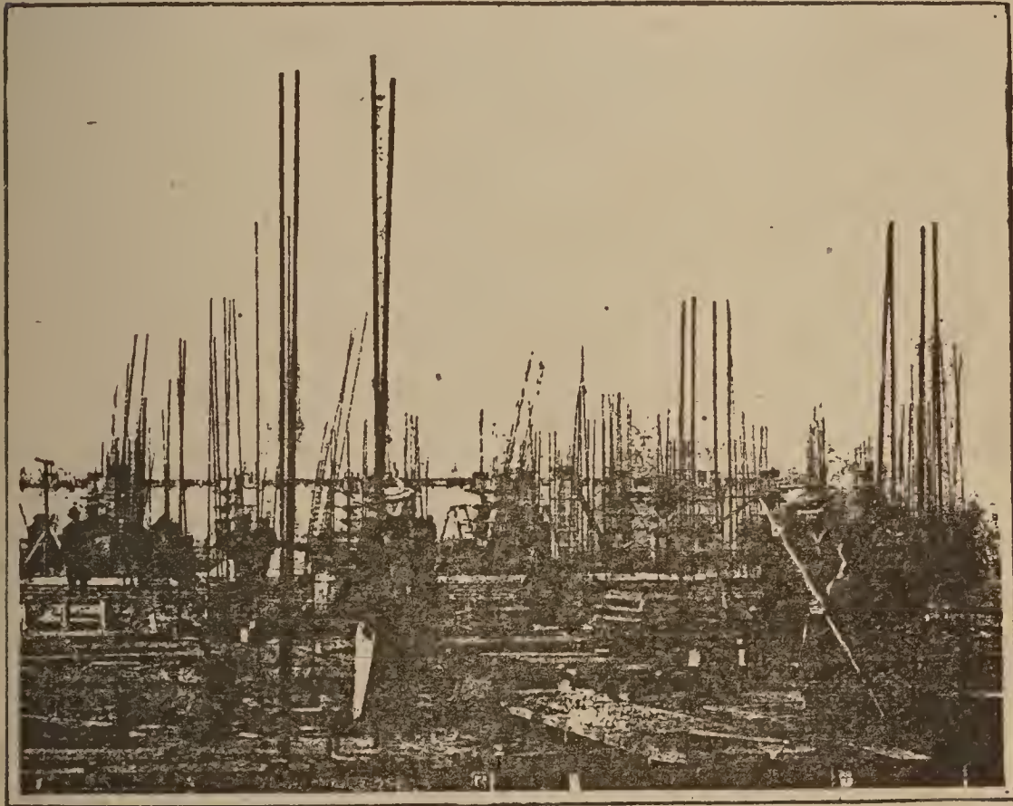
Fig. 7.—Ransome System of Erecting Columns.
