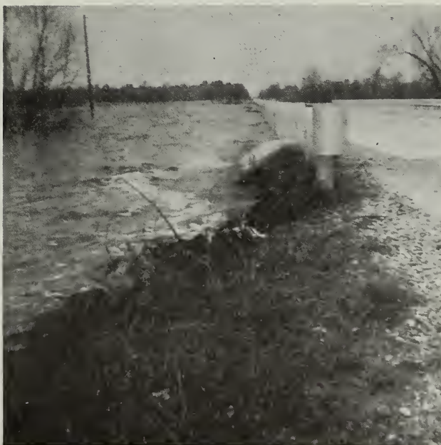
Flooding of Sumter County Highway 21 bridge over Factory Creek
