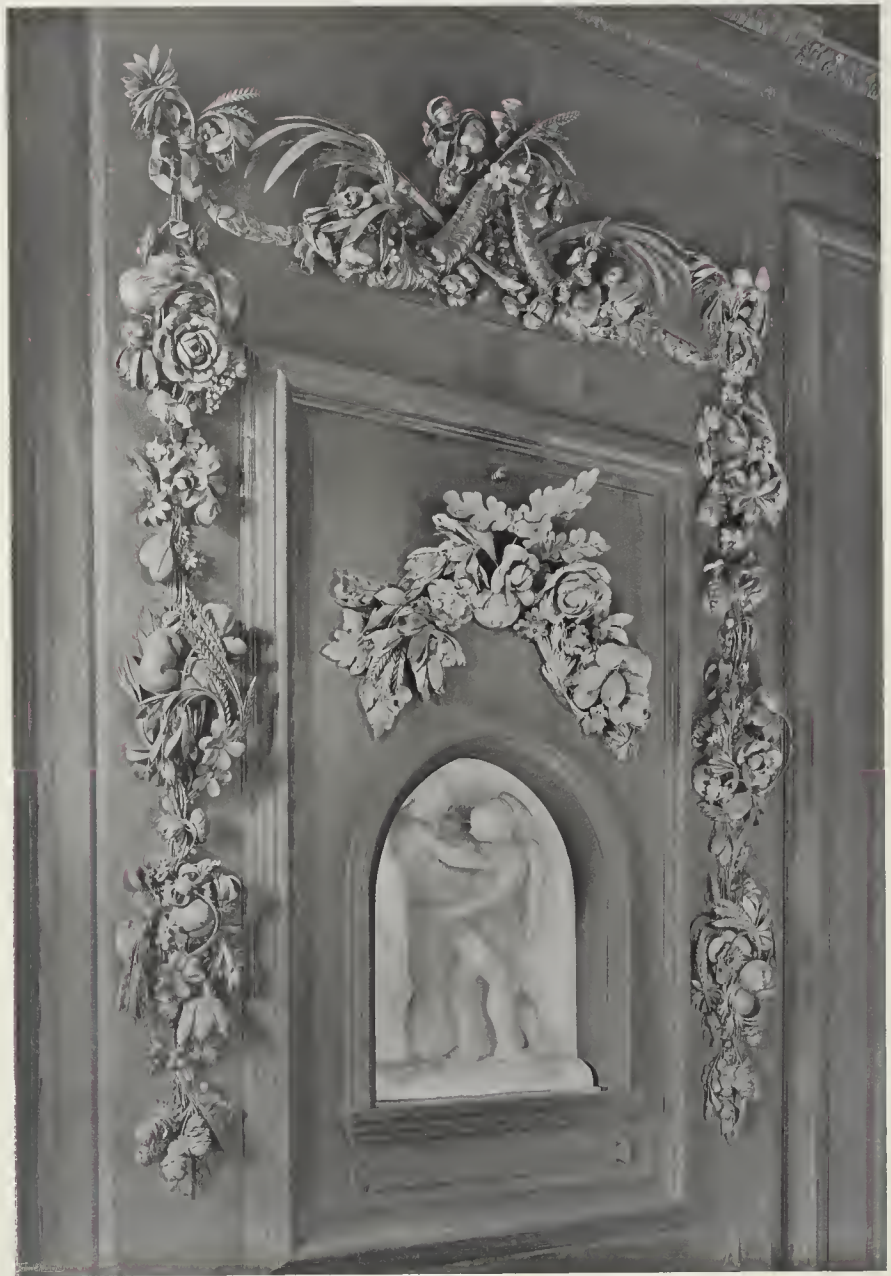
FIG. 192.—BELTON : OVER THE CHIMNEY-PIECE OF THE CHAPEL GALLERY.
