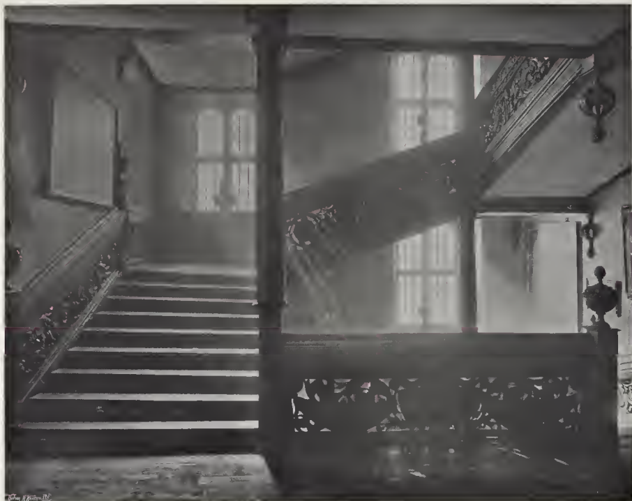
FIG. 27.—STAIRCASE, DURHAM CASTLE.
