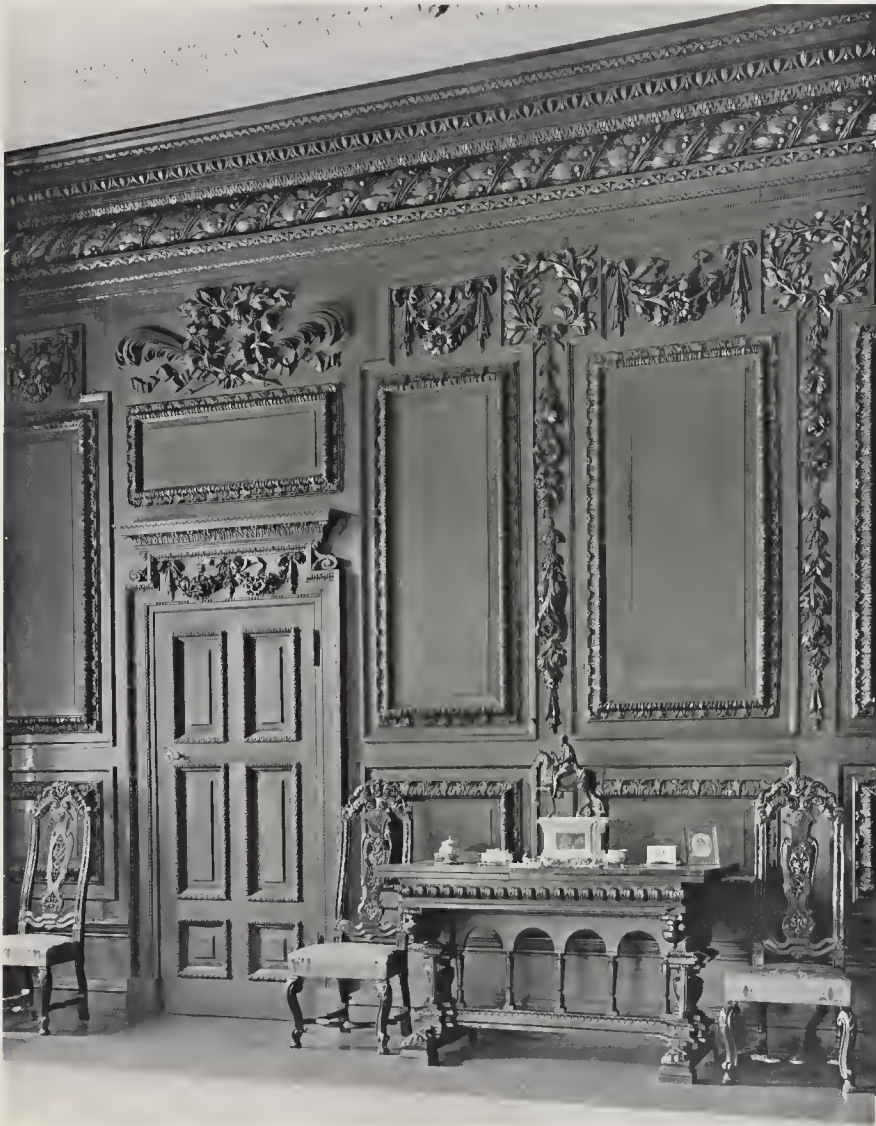
FIG. 222.—HURSLEY: DOORWAY AND PANELLING IN THE HALL.
