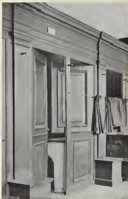
FIG. 172.—A CUBICLE, CHELSEA HOSPITAL.
