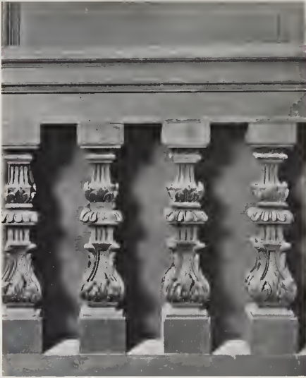
FIG. 94.—DERELICT BALUSTERS FROM GALLERY.
