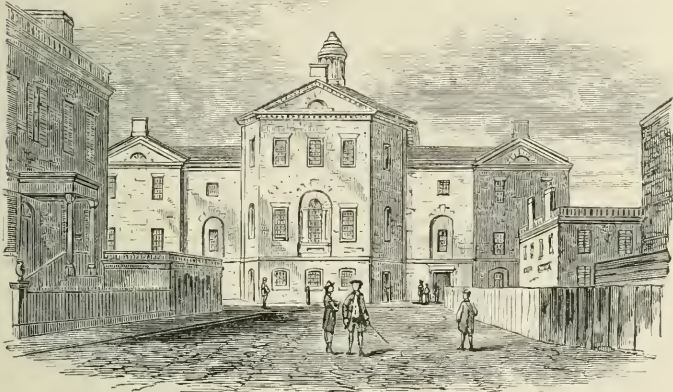
THE OLD COURT HOUSE AND CITY HALL.
