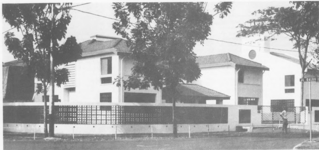
JAKARTA, Indonesia —This is 1 of 14 recently-completed staff housing units, each having three or four bedrooms and its own carport. The houses are constructed of stucco over masonry and are air-conditioned.
