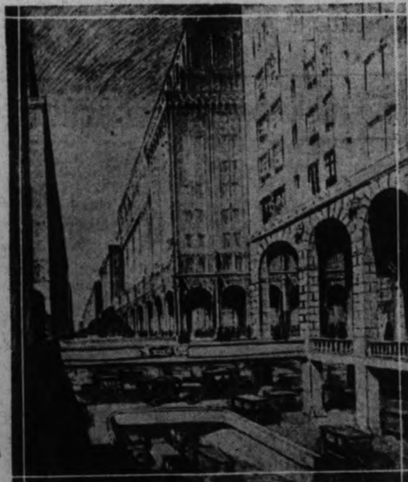
THEY'RE COMING TO THIS IN N.Y. —Under proposed triple deck street plan New York street crossings will one day be bridged in all directions; an upper level for pedestrians; crosstown traffic and vehicular traffic would pass on the lower levels.
