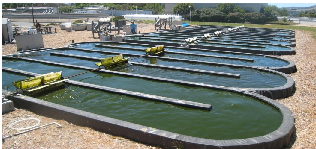
Fig. 7. Use of Algae pounds for water purification.
