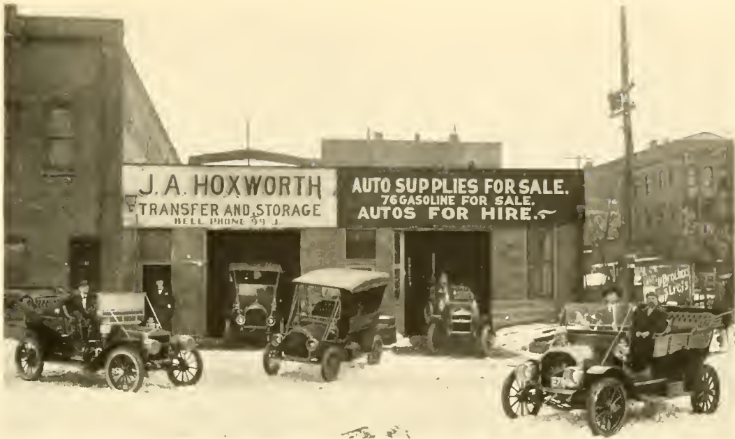
J. A. HOXWORTH TRANSFER AND STORAGE OFFICE AND GARAGE, CANONSBURG
