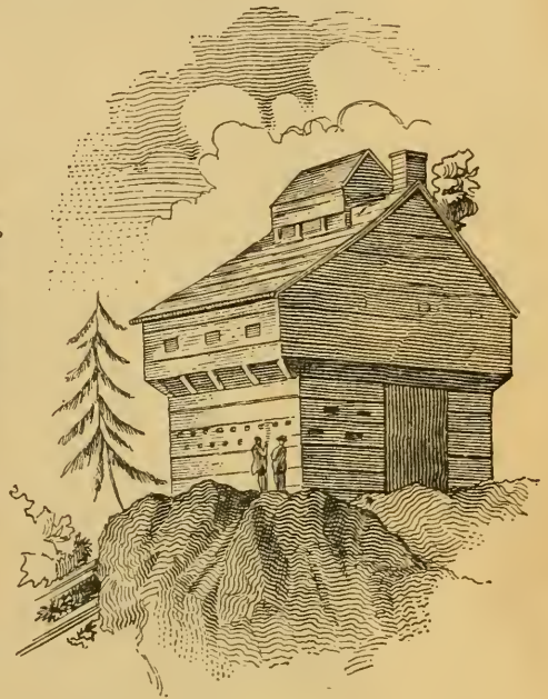
A Block House, Exterior
