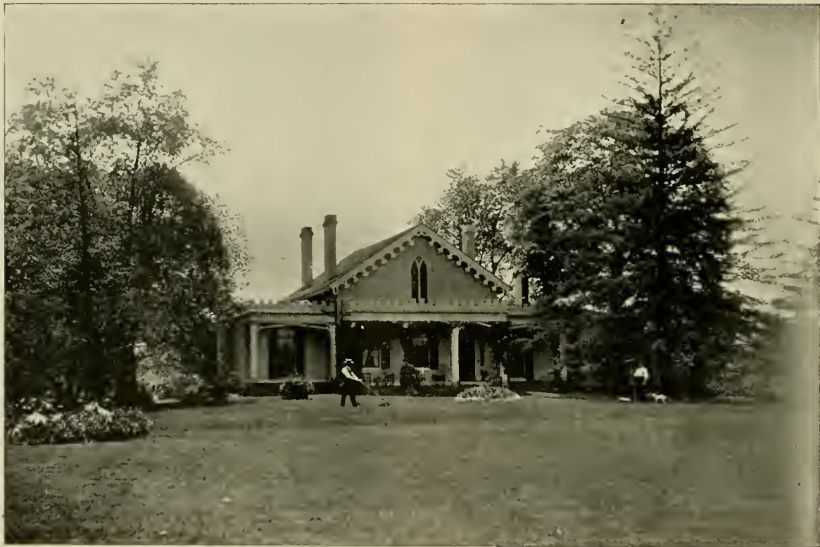
RESIDENCE OF MRS. THOMAS BOLTON. (Built 1846.)
