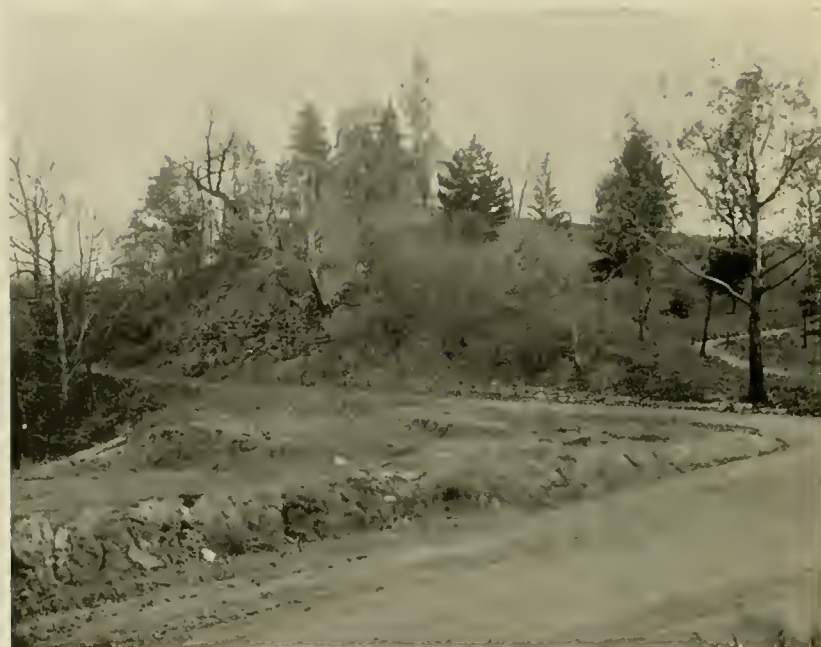
ENTRANCE TO VINECLIFF—AMBLER PARKWAY.
