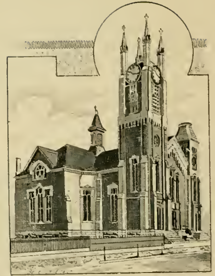
FIRST CONGREGATIONAL CHURCH. (Akron.)
