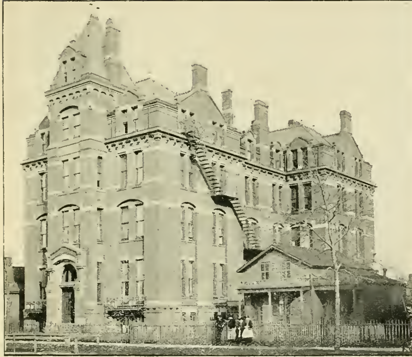
HURON STREET HOSPITAL.
