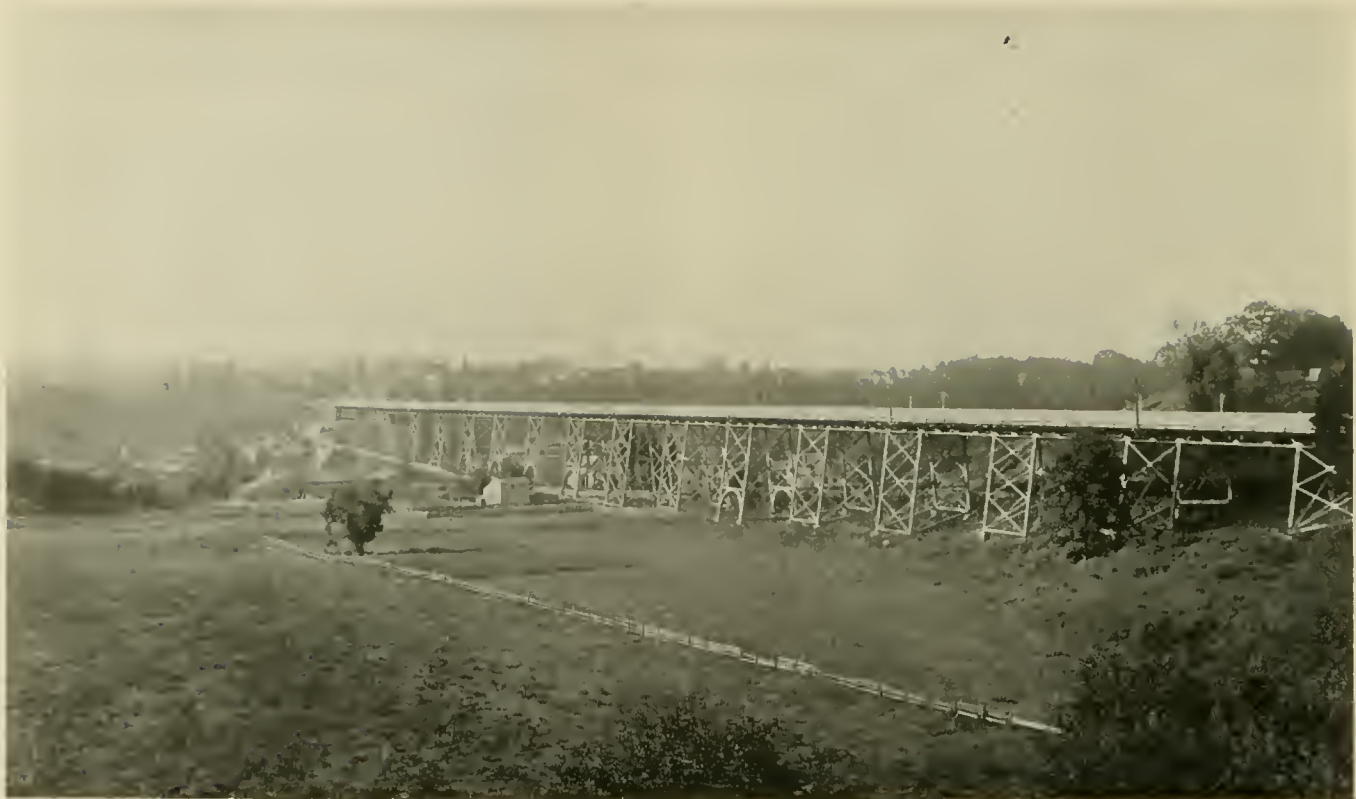
VIADUCT AT ENTRANCE BROOKLYN PARK.
