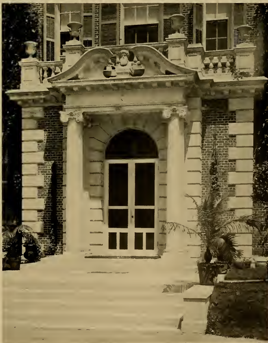
THE MAIN DOORWAY.
