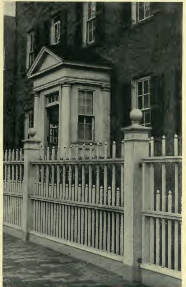
FENCE DETAIL House in Newburyport, Massachusetts
