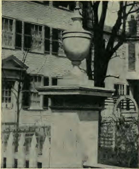
FENCE POST, NEWBURYPORT, MASSACHUSETTS
