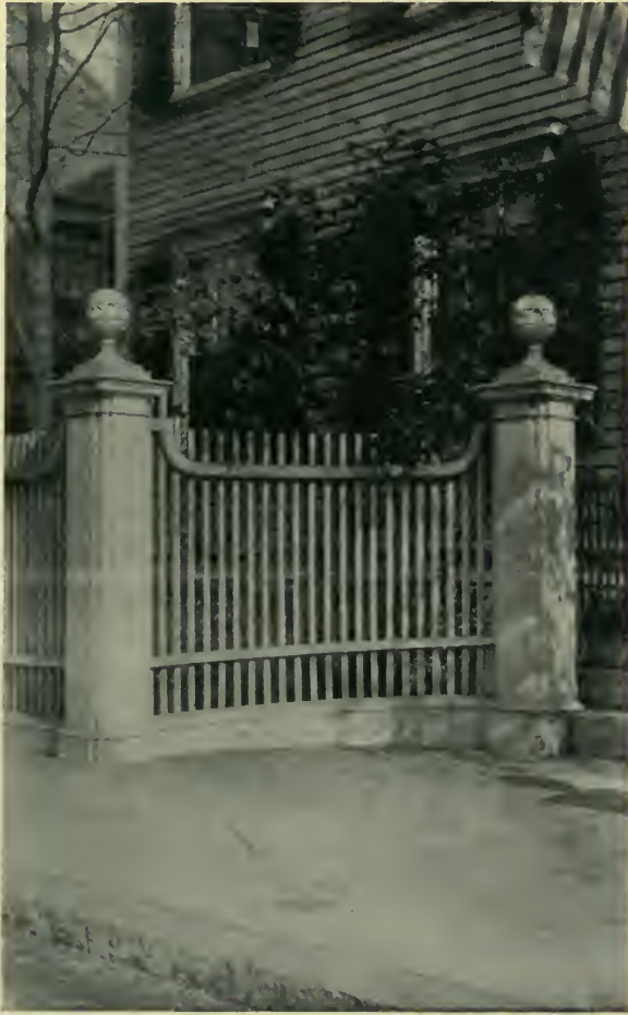
FENCE DETAIL House in Newburyport, Massachusetts
