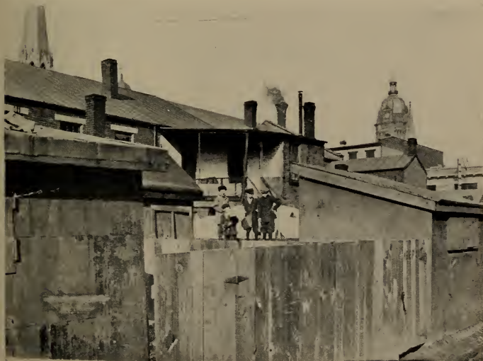
No. 1, front of tenement row; dark, damp and unsanitary No. 2, rear of same, No playground but street, alleys, ashbins and sheds
