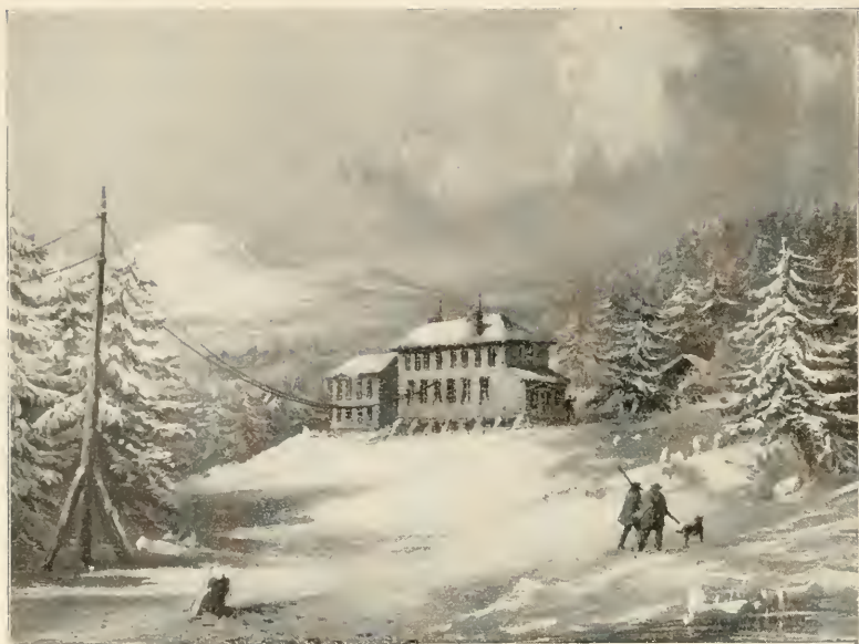
TRINITY BAY, NEWFOUNDLAND. EXTERIOR VIEW OF THE TELEGRAPH HOUSE IN 1857-1858.
