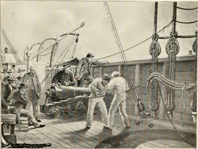
SPLICING THE CABLE AFTER THE FIRST ACCIDENT ON BOARD THE GREAT EASTERN.
