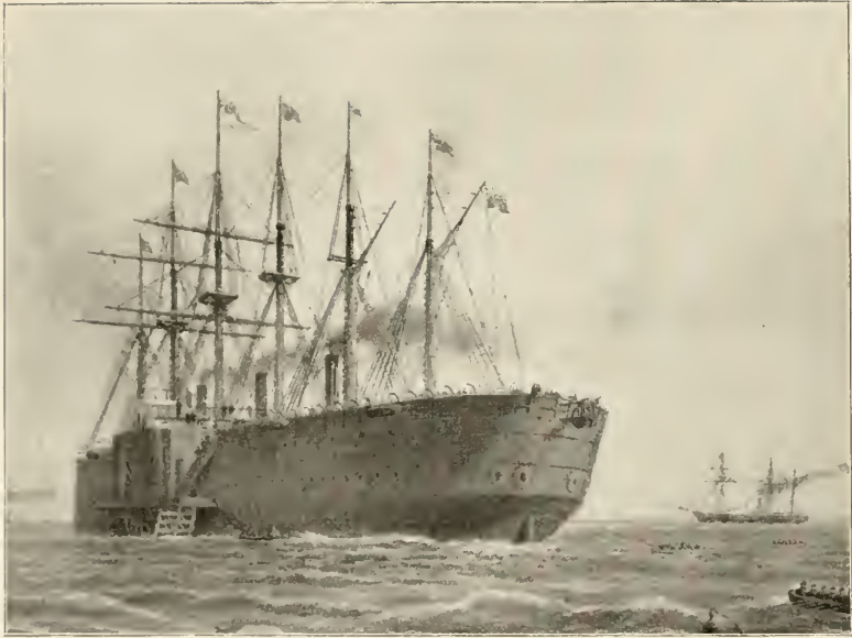
THE GREAT EASTERN UNDER WEIGH, LAYING THE CABLE.
