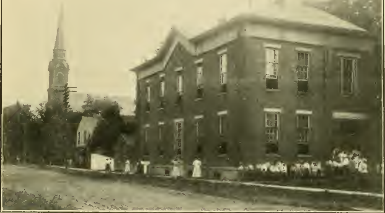
VEVAY HIGH SCHOOL BUILDING Undergoing Extensive Repairs At Present
